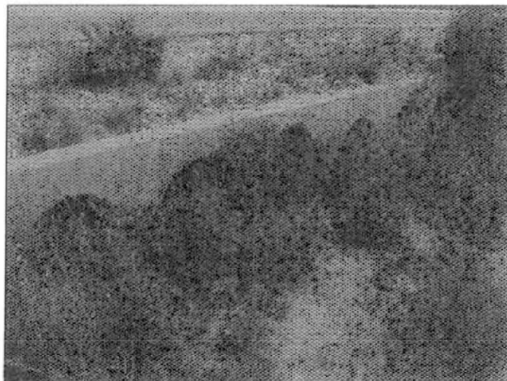
6 - 29" x 18" CMP ARCH CULVERTS UNDER THE ACCESS ROAD
