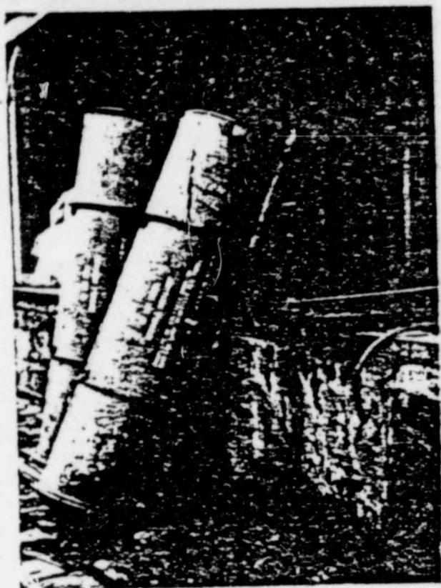
FIG. 21 OLD PRODC SHIPPING CONTAINER USED FOR WATER DRUM.
