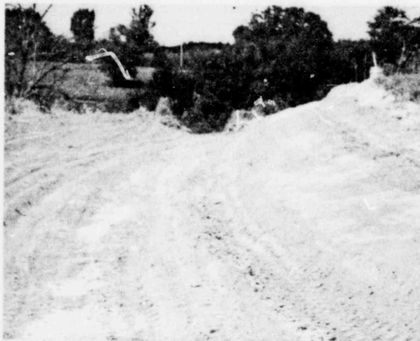
FIGURE 49 : DDC-1; looking north from the red flagged stake at the right side of the channel bend shown in Fig. 48.
