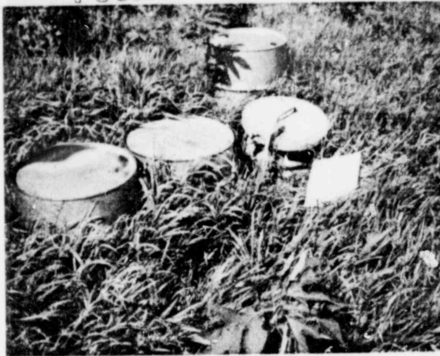
FIGURE 3 : Three corrugated metal pipe piles, capped with concrete lids and covered by steel drums; located near 12347N/14470E.
