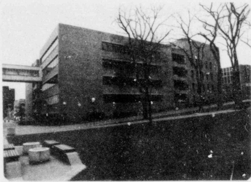
CRAMER HALL VIEW: SOUTHEAST
