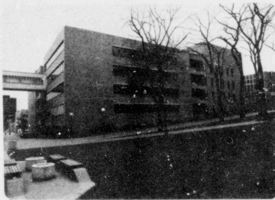
CRAMER HALL VIEW: SOUTHEAST
