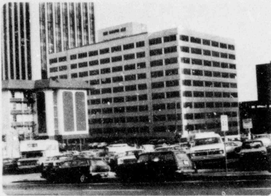
STATE OFFICE BUILDING VIEW: EAST
