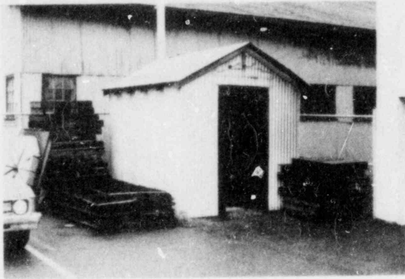
HIGHWAY TEST LAB INSTRUMENT SHELTER VIEW: NORTHEAST
