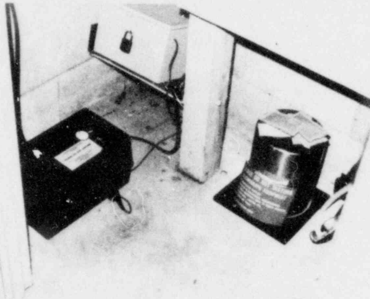
SMA-1 Accelerograph Rectifier/Control Building
