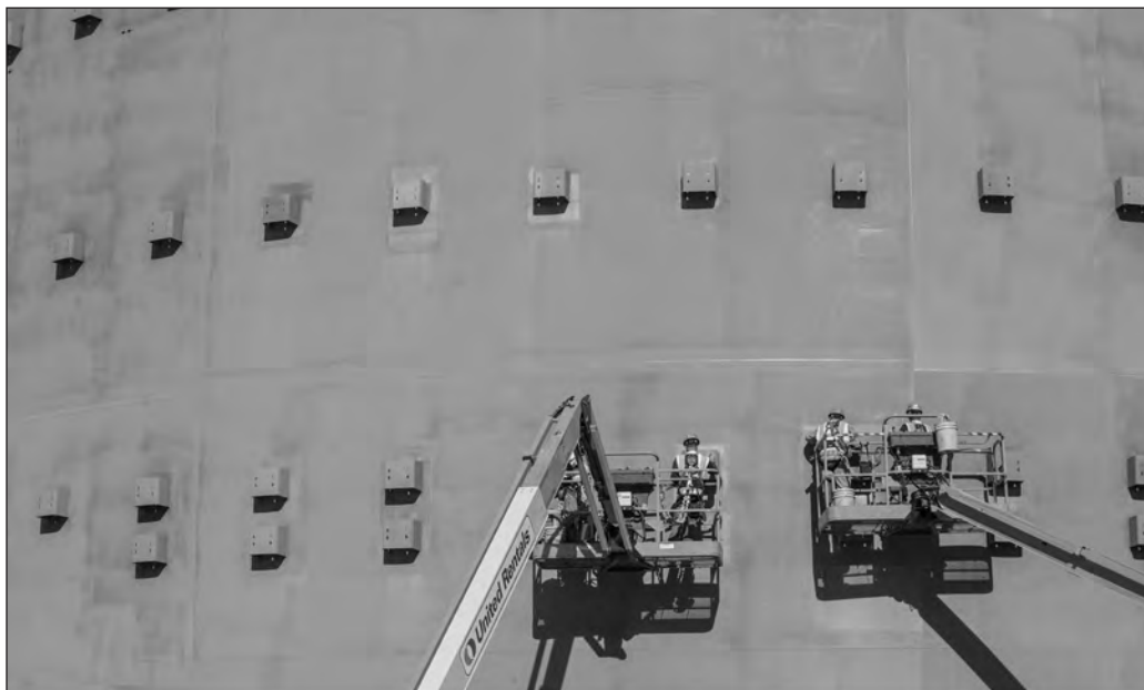
Vogtle Unit 3 middle ring. Photo courtesy of George Power Company.
