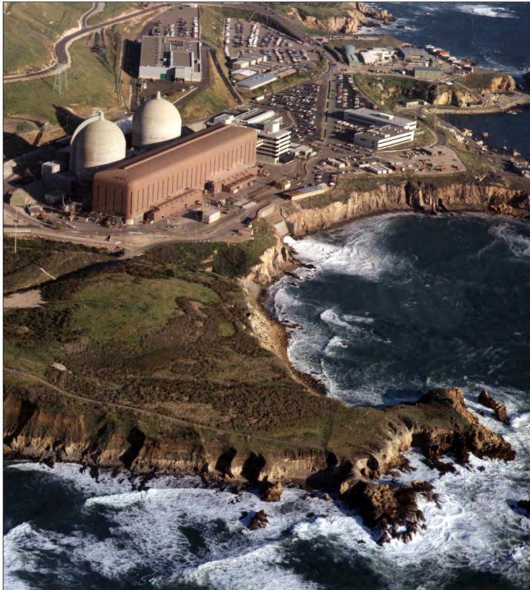
Diablo Canyon Nuclear Power Plant, Units 1 and 2.
