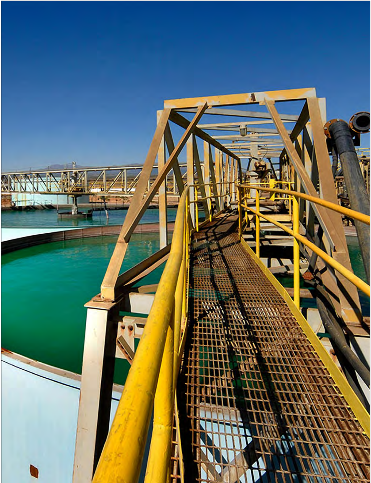
The White Mesa uranium mill is located in Blanding, Utah, near the uranium mines of the Four Corners region of the United States. Energy Fuels, Inc. constructed the mill in 1980. The mill uses sulfuric acid and a solvent to extract uranium and vanadium. Courtesy of Energy Fuels, Inc.
