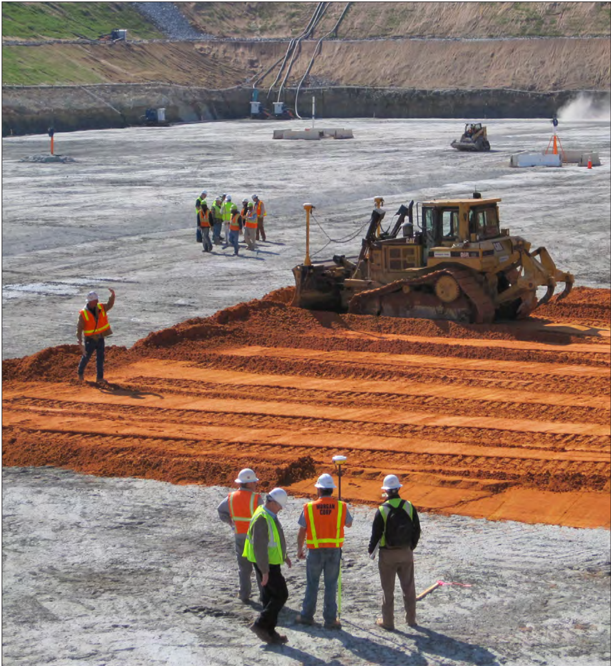
Backfill begins on Vogtle Unit 3. Courtesy of Southern Nuclear.
