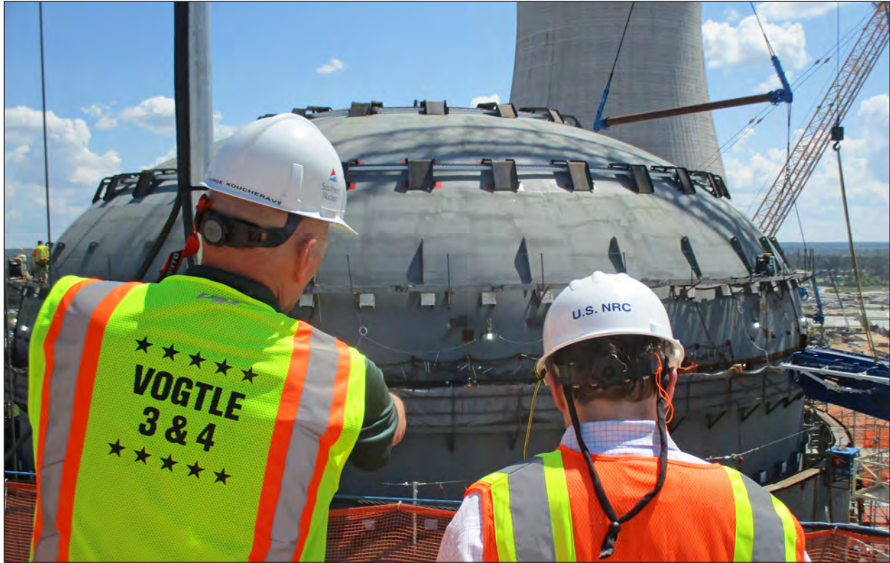
NRC Commissioner Jeff Baran (right), with Southern Nuclear's George Koucheravy, got a bird's-eye view of the containment building under construction during a recent visit to the Vogtle 3 & 4 construction site in Waynesboro, Ga.
