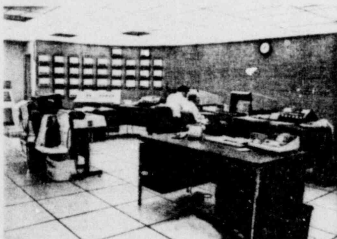
Overall coordination of the Dairyland Power System is accomplished at the Operations Control Center located in the general office building at La Crosse. It is here that decisions are made which correlate the operation of generating sources, the transfer of bulk power to and from neighboring systems and transmission network switching in order to achieve optimum economy, stability and security.
