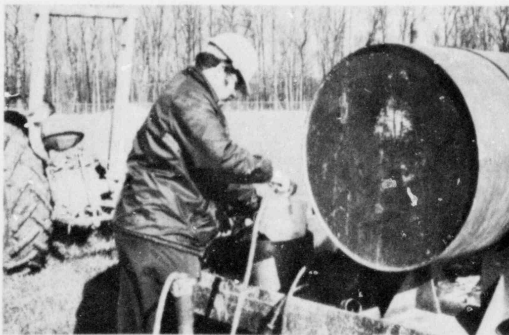
Figure 3.1. Portable unit used for pumping water from trenches at Maxey Flats.
