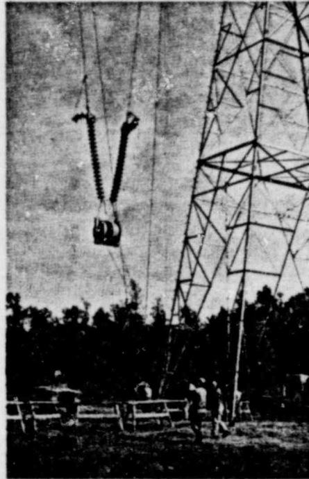
At the close of 1966, the Company's 345-mile, 500,000-volt transmission system was near completion. The lines are part of the nation's largest Extra High Voltage system.
