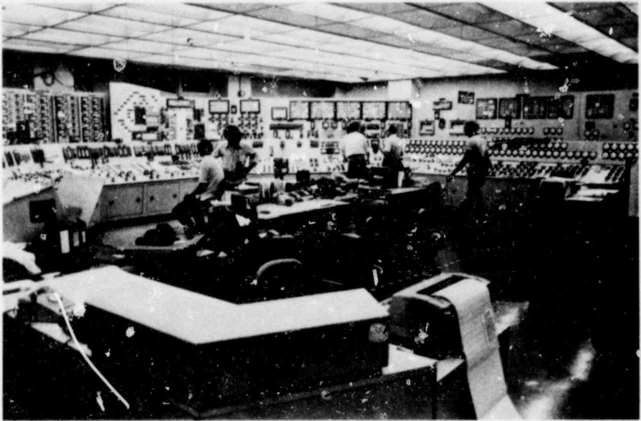
FIGURE II-48. TMI Control Room (Postaccident)
