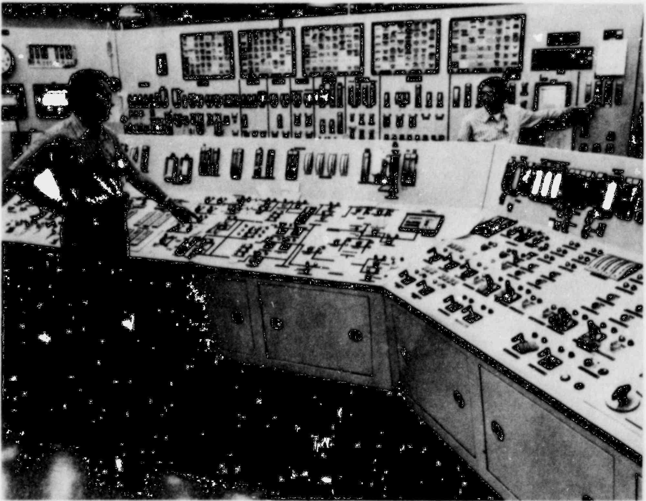
FIGURE II-49. Visual Scan Necessary for Operator (on Left) Controlling Makeup To Monitor Makeup Flow (Operator on Right)
