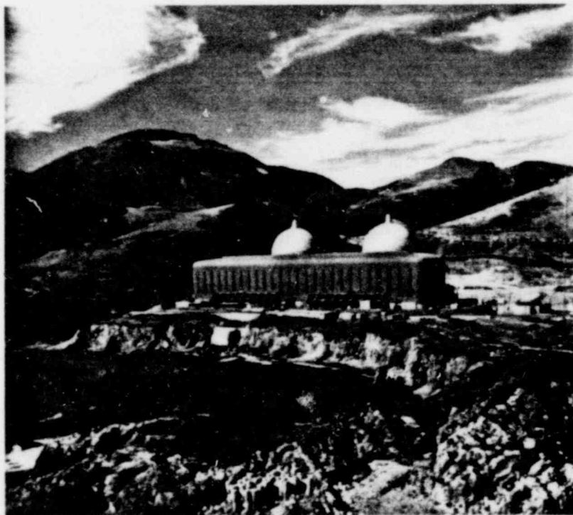
PG&E's 2,200,000 kilowatt Diablo Canyon Nuclear Power Plant is located on an isolated stretch of the Central California coastline.
