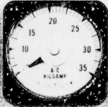
GENERATOR AMPS AC
