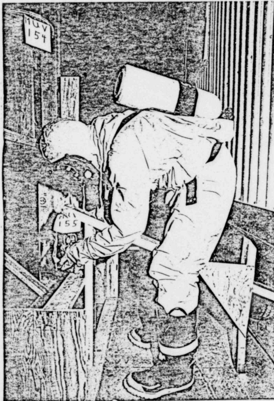
TIGHTENING PACKING ON MU-V-155
