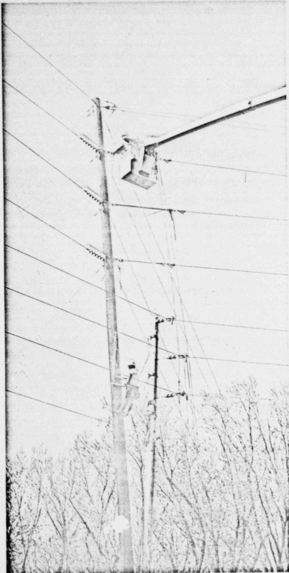
Dairyland Power Construction crews work on the four-mile N-149 line (69 kV Albion Tap off a Northern States Power Co. line) in Wisconsin near Black River Falls. This line was energized June 28, 1979.
