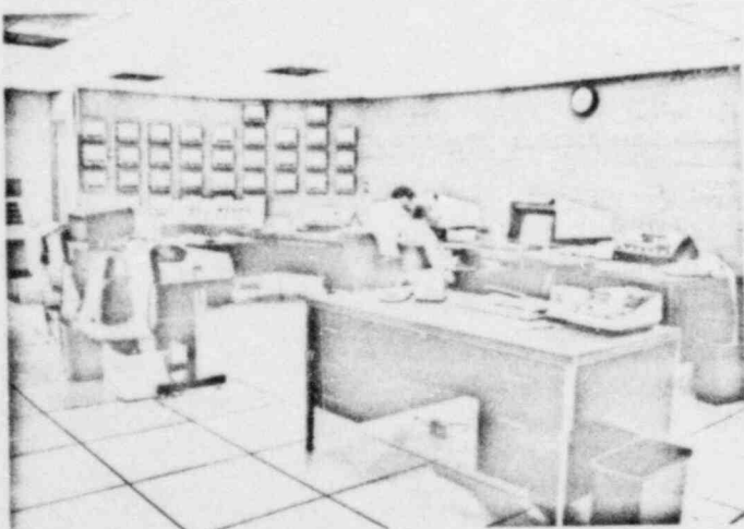
Overall coordination of the Dairyland Power System is accomplished at the Operations Control Center located in the general office building at La Crosse. It is here that decisions are made which correlate the operation of generating sources, the transfer of bulk power to and from neighboring systems and transmission network switching in order to achieve optimum economy, stability and security.
