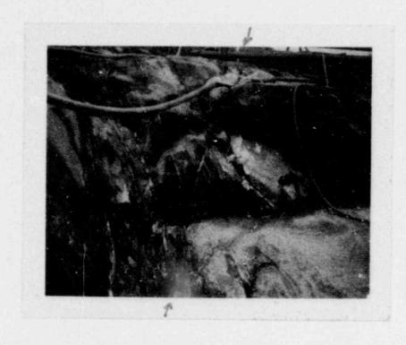
View East. Fault located on north end of spent fuel storage pool - Unit 2 Fuel Building. Approximately 106 feet north of east-west baseline.
