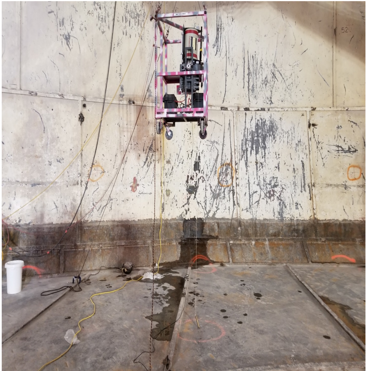
Figure 11 - ISOCS Measurements of Unit 2 Containment Above 565 foot Elevation
