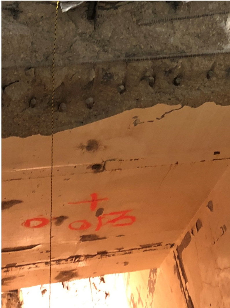
Figure 10 - Unit 2 Under Vessel Incore Tunnel Remediation
