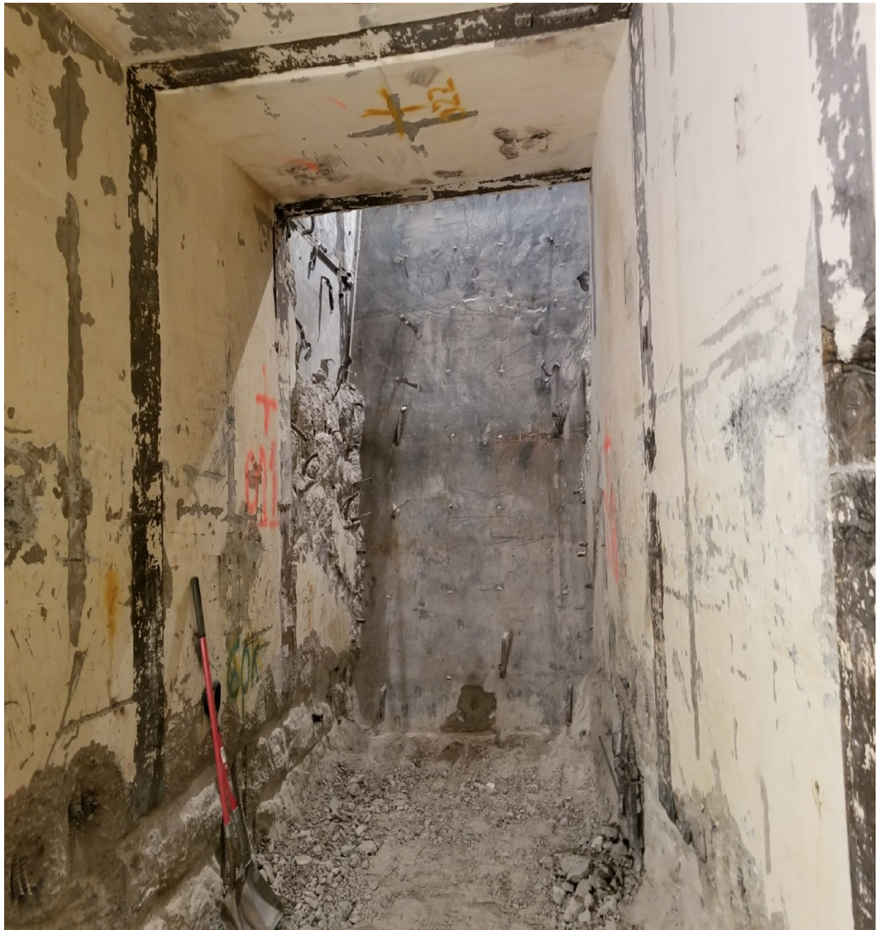
Figure 4 - Unit 2 Containment Incore Tunnel
