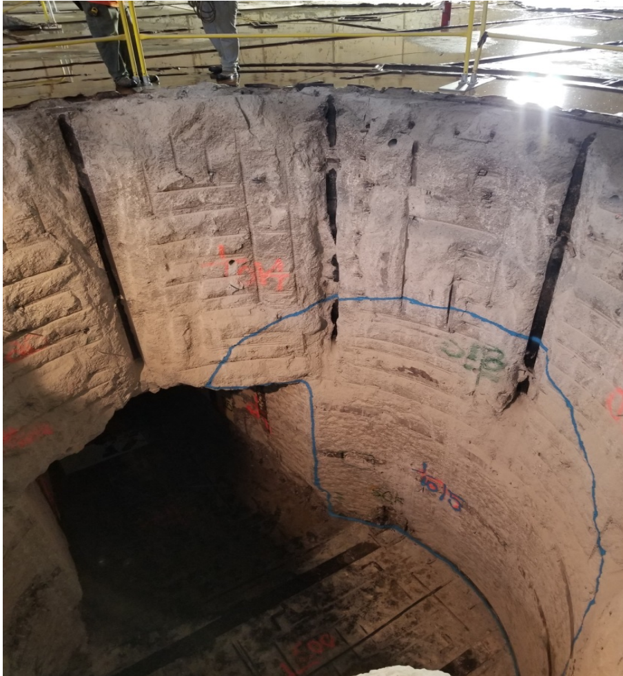
Figure 14 - Unit 2 Under Vessel Concrete H-3 Concrete Remediation Area
