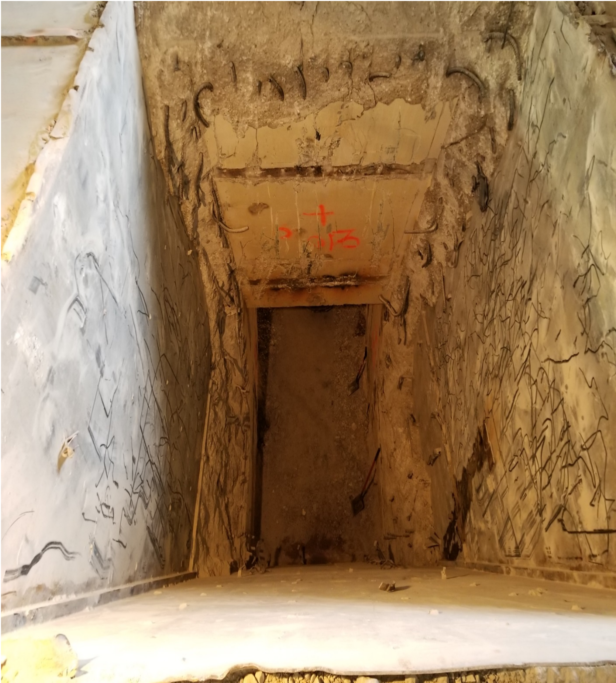
Figure 5 - Unit 2 Containment Sloped Tunnel
