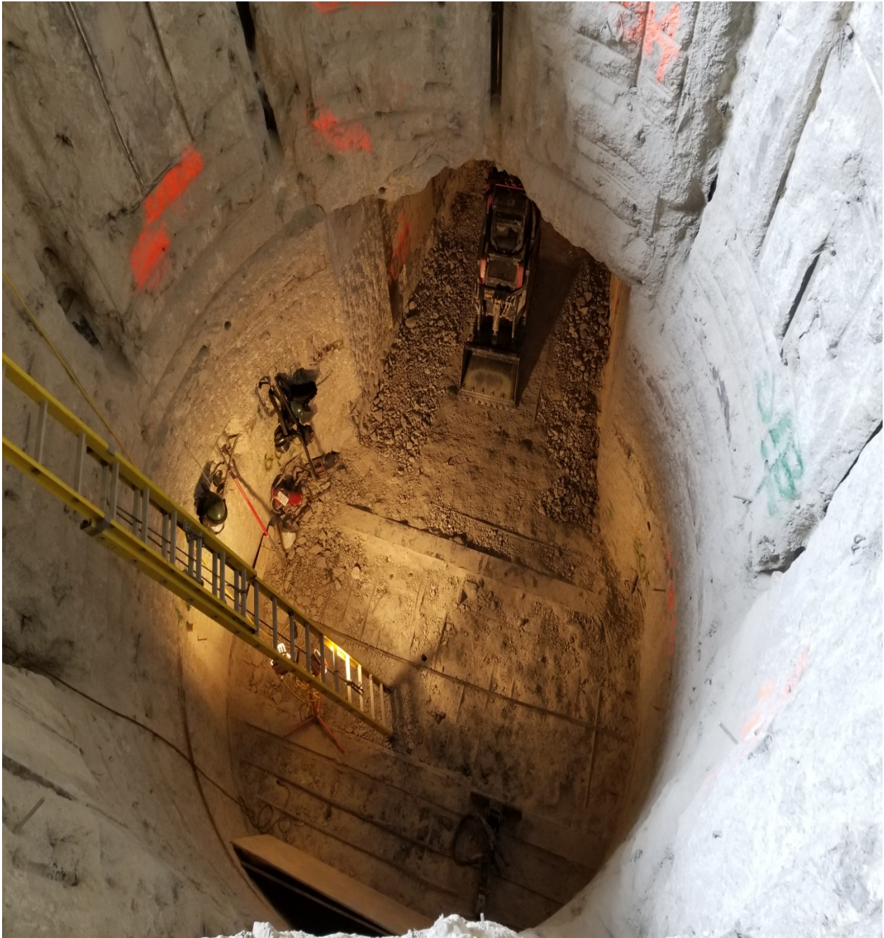
Figure 3 - Unit 2 Containment Under Vessel
