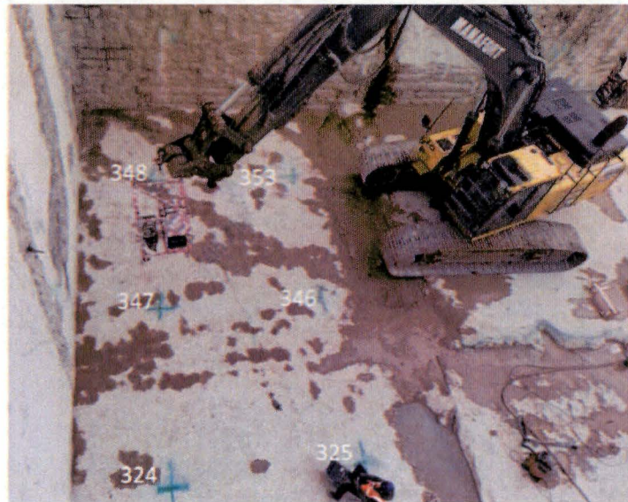
Figure 4-1 – ISOCS Systematic Measurements of Auxiliary Building 542 foot Elevation
