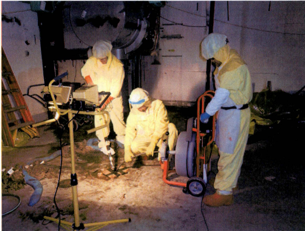
Figure 3-3 – Embedded Drain Pipe FSS Survey
