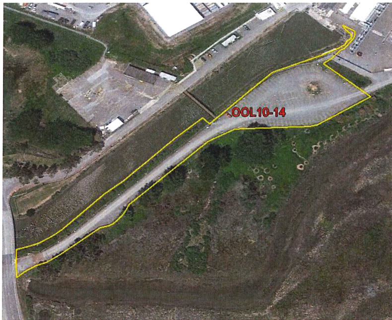
Figure 1.5 - Phase Release Area of OOL10-14
