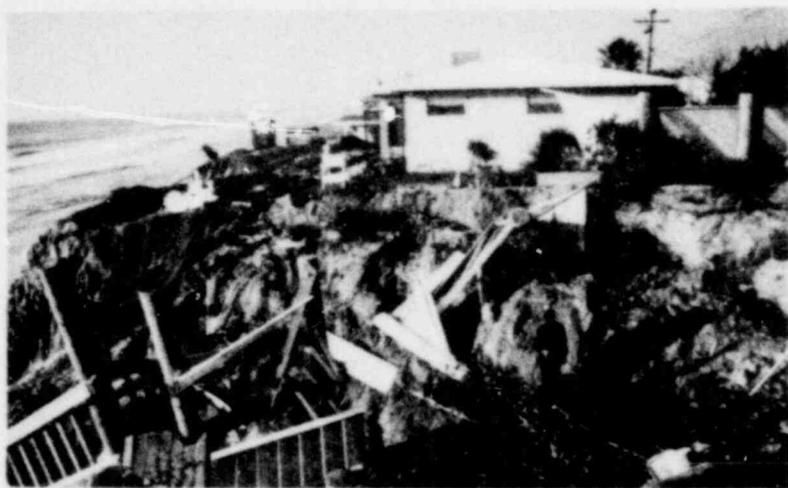
Figure 5A. View northeast shows stairway at D Street, Encinitas. It collapsed, starting at the top, during the rains of January, 1978.
