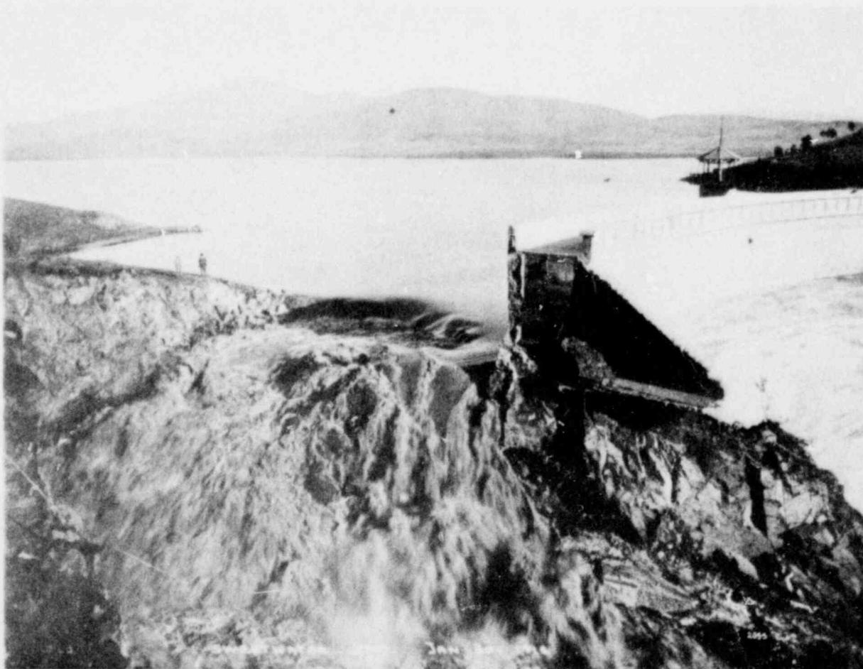
Figure 1. Water flowing through breached abutments of Sweetwater Dam, January 30, 1916.
