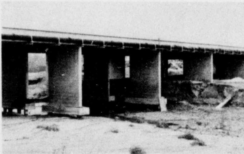
Figure 4. Stream-bed erosion in the San Diego River channel at the Magnolia Avenue bridge across the San Diego River in Santee. Erosion has exposed both pile caps and piles.
