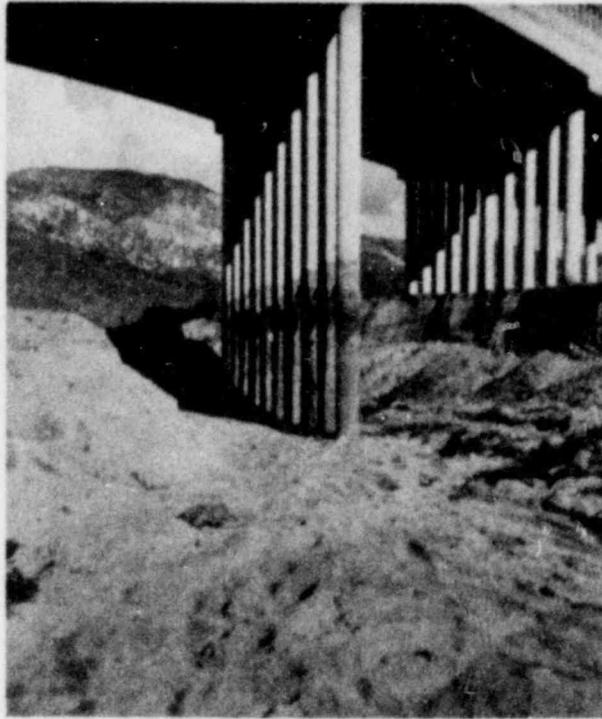
Figure 3. Stream-bed erosion in the San Diego River channel at the Highway 67 bridge over the San Diego River north of Lakeside. Approximately 10 feet (3 m) of erosion has connected deep, sand borrow pits on either side of the bridge.
