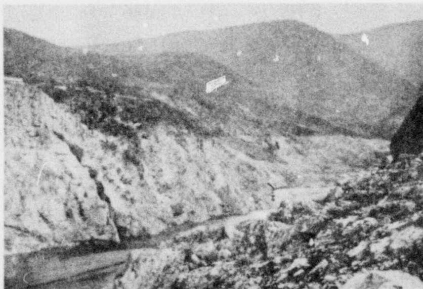
Figure 3. Lower Otay River valley after failure of the dam. Note dam abutment near lower left corner and valley walls cleansed of soil and vegetation by the flood water.
