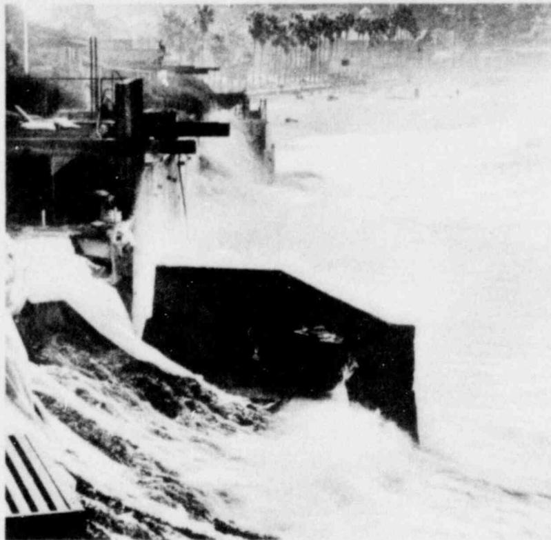
Figure 3. Storm waves battering homes along alluvial cliffs south of Scripps Institution of Oceanography, looking south. A section of the concrete seawall in the foreground collapsed later. M. Clark photo, S.I.O., February 7, 1978.
