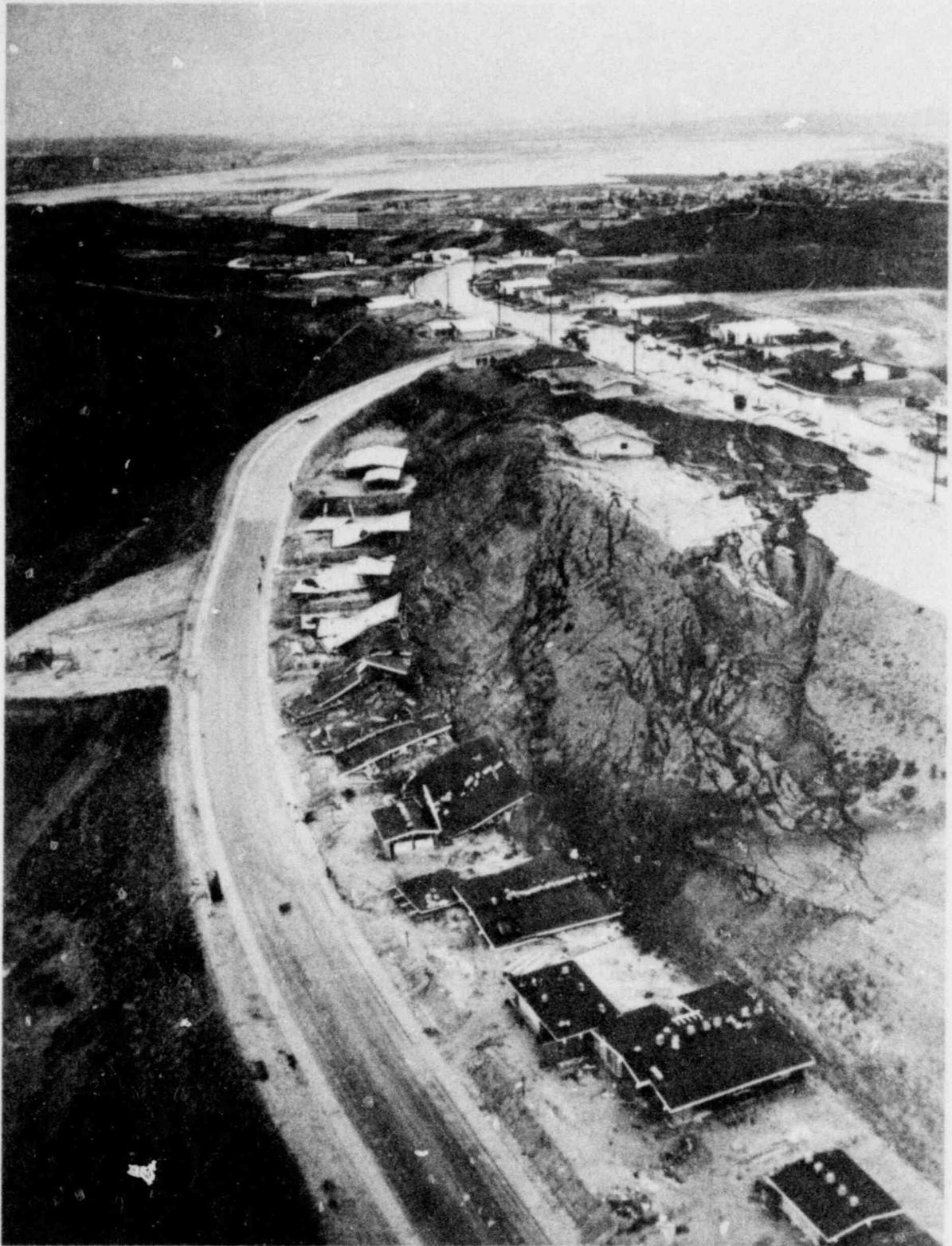
Figure 1. View of Mount Soledad landslide of December 14, 1961, looking toward the south. Landslide destroyed seven homes under construction near the intersection of Desert View Drive and Soledad Mountain Road. Failure was due principally to oversteepening of faulted and jointed, Eocene Ardath Shale inclined in the same general direction as the cut slope. Photograph from Union-Tribune Publishing Co., San Diego, CA.
