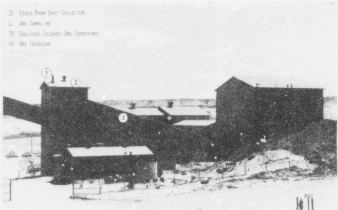
Figure 5.7 Structures Housing Ore Crushing Operations (Note absence of these structures in a new mill shown in Figure 5.4 which utilizes wet-semiautogenous grinding (SAG) of ore. The SAG process eliminates dry crushing of ore; see Figure 8.1.)
