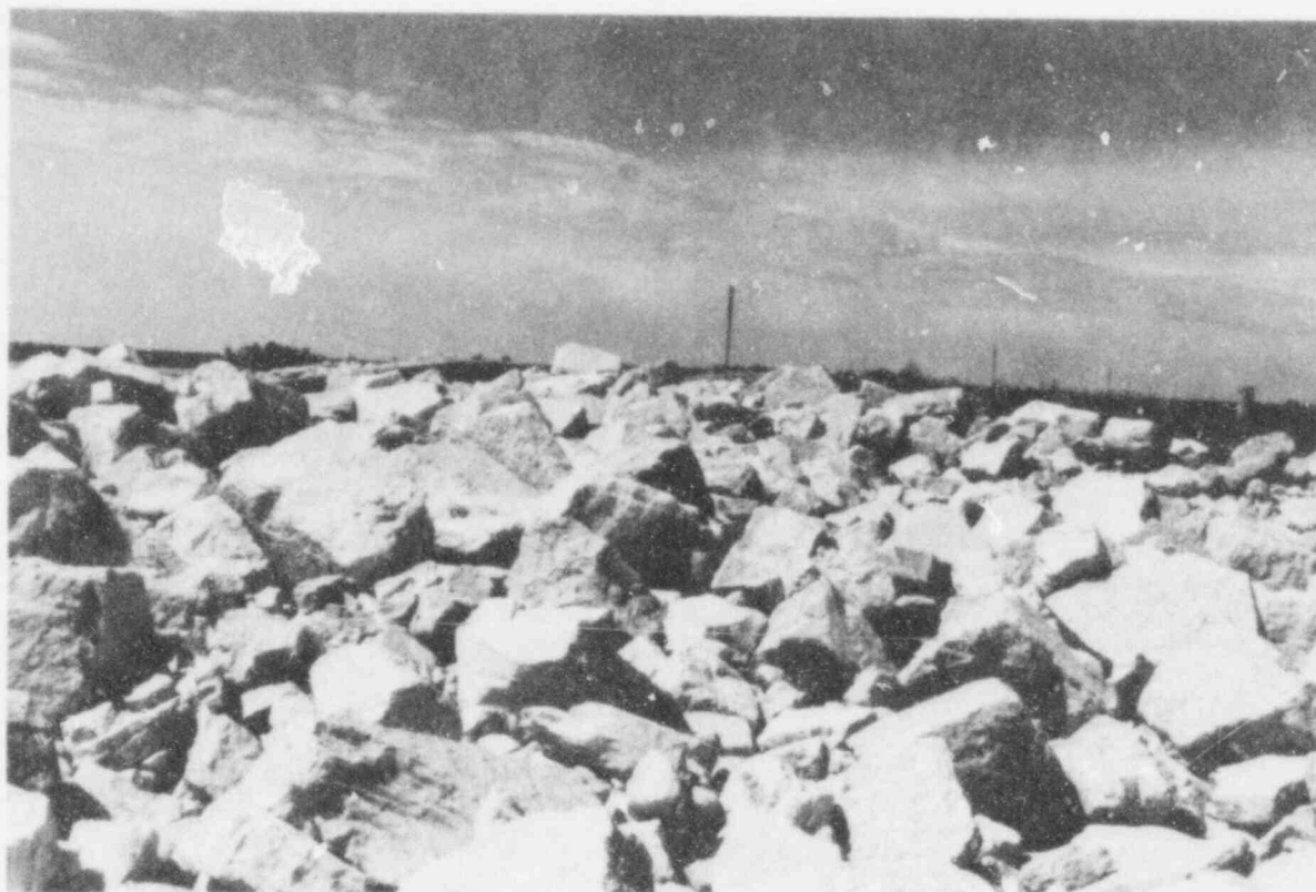
Figure 8.3 RIP RAP COVER ON EMBANKMENT SLOPE
