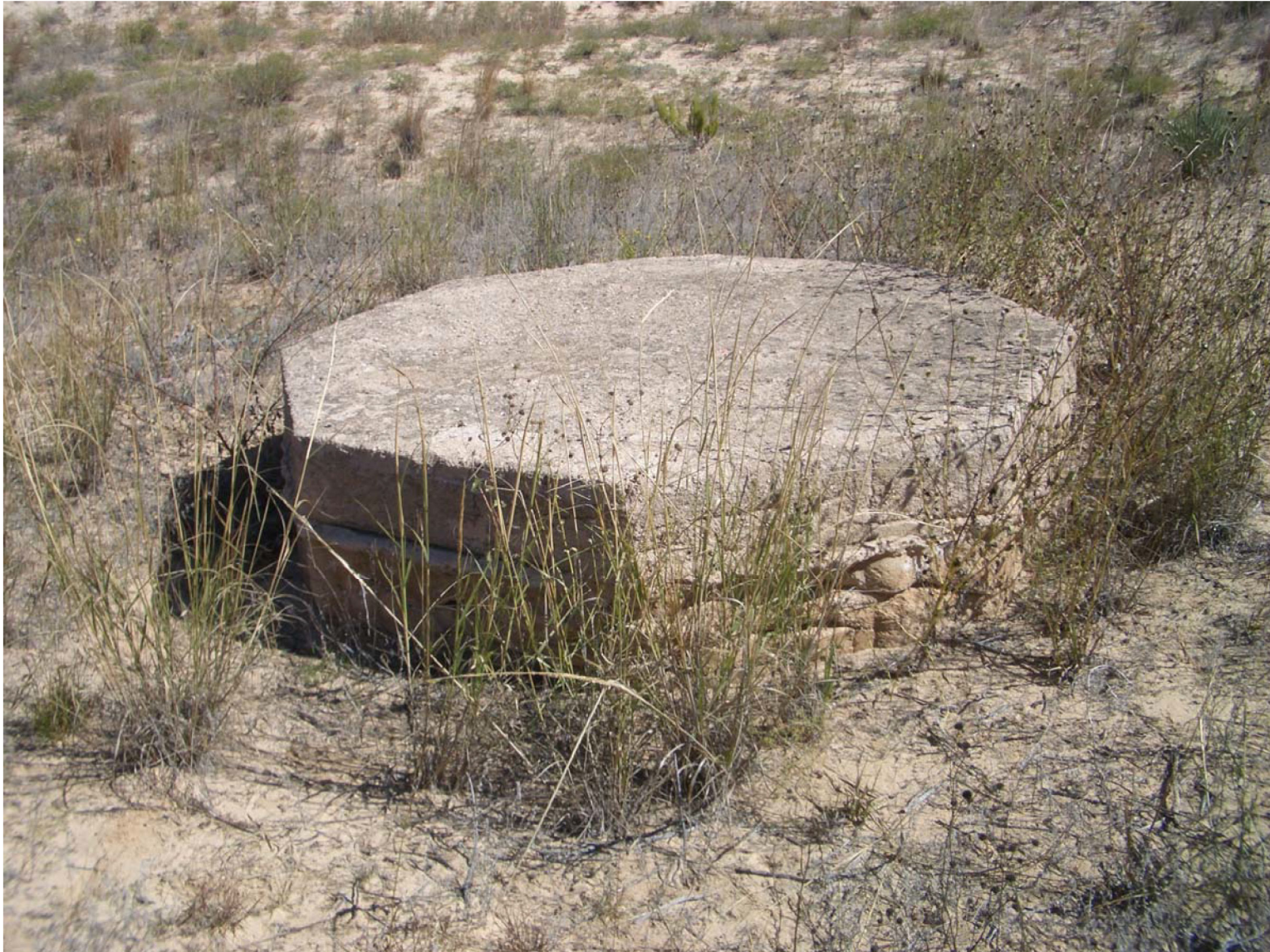
Figure 15 - Location #9, Looking Northeast
