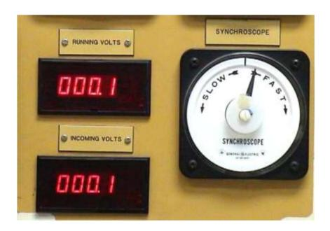
**Answer:** A (1) frequency (2) Main Generator frequency is higher than switchyard frequency
