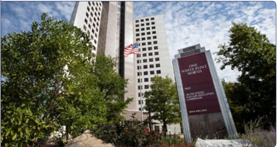
The NRC Headquarters complex is located in Rockville, MD.
