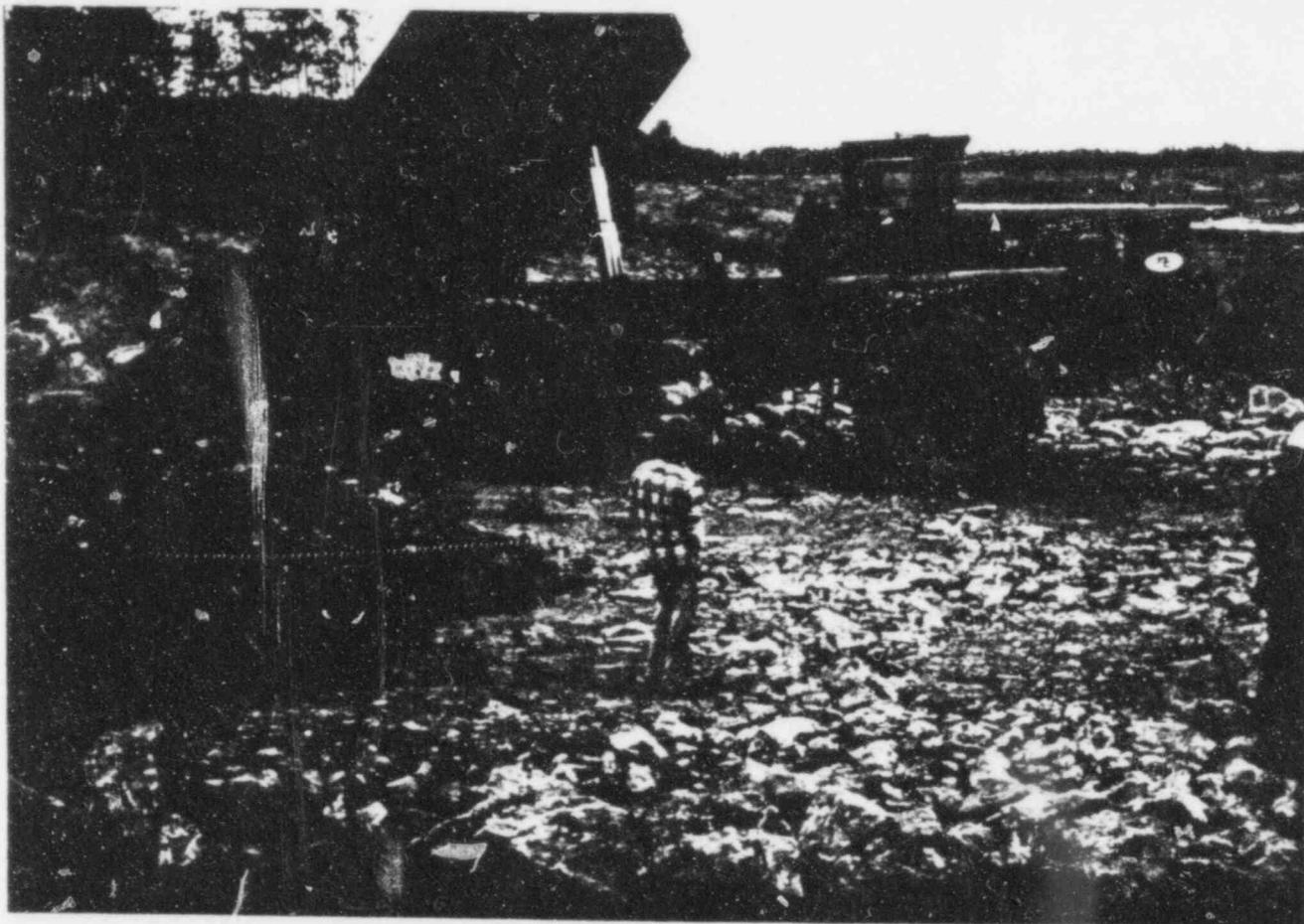
Photo 2 End dumping of Rock on Test Section V.P. 1D 24-4-3. **POOR ORIGINAL**
