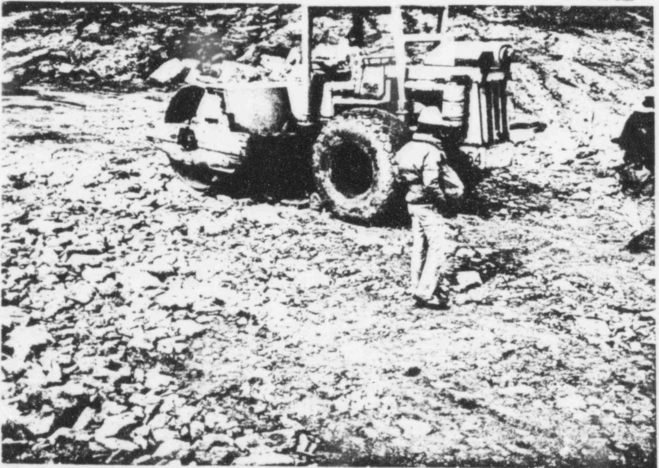
Photo 5 Test Section VRMD-24-4-3 during rolling with smooth drum vibratory roller.
