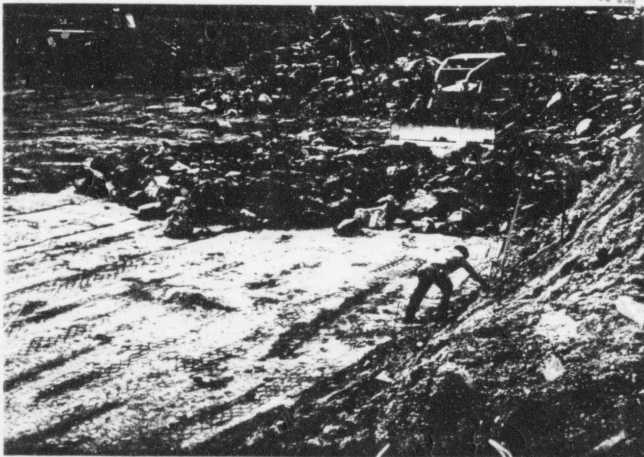
Photo 3 Spreading of Rock to 24 inch nominal lift thickness with dozer. 496 243
