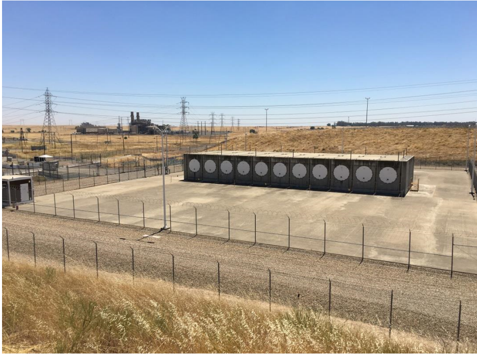
Figure 1.3: Rancho Seco ISFSI Horizontal Storage Modules (SMUD, 2018)
