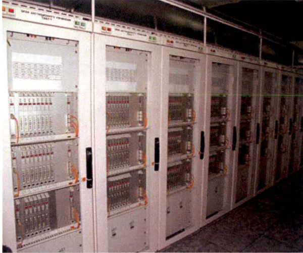
Eighteen ESFASs are presently in operation at Rivne, South Ukraine, and Kozloduy (Bulgaria) NPPs.
