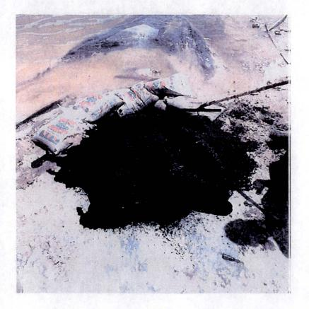
Photograph 2: View showing liner after repair with fabric patch and sealed with Deery Oil #6
