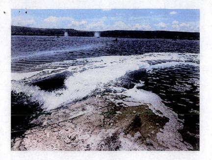
Photograph 1: View showing water discharge causing water/air to infiltrate below liner
