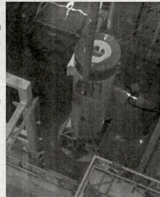
Lifting operation for irradiated materials transport cask
