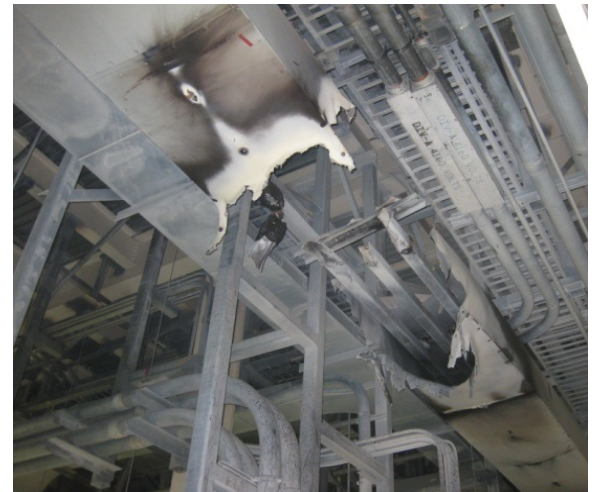
Columbia Bus Duct (OpE) 2009
