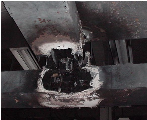
Diablo Canyon Bus Duct (OpE) 2000
