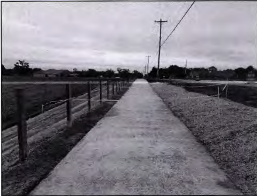
Photograph 1: Area where the Cesium 137 source was found underneath the concrete (5/21/2019).
