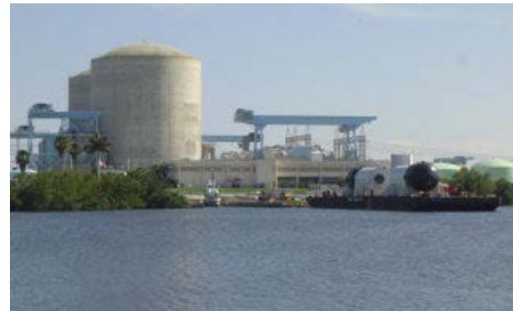
St Lucie Nuclear Power Plant.
