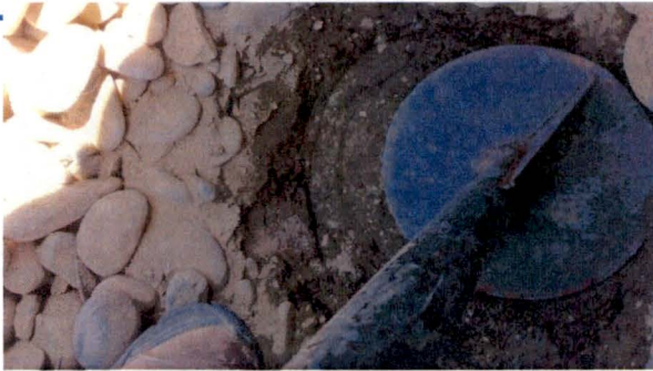
Photograph 12. Near Surface Compaction Tool Used
