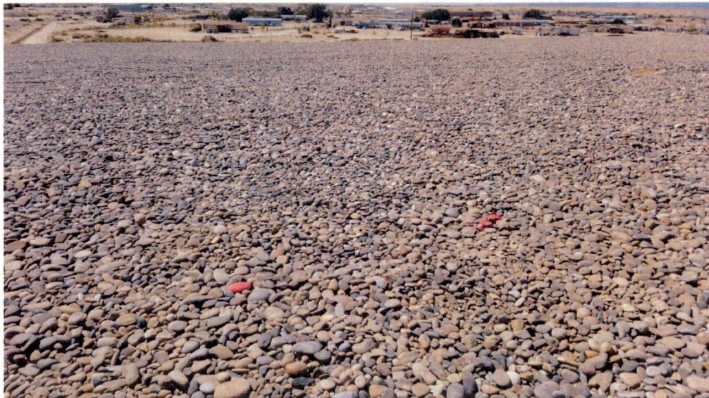
Photograph 16. Final Surface at Location 205
