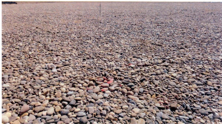
Photograph 19. Final Surface at Location 208
