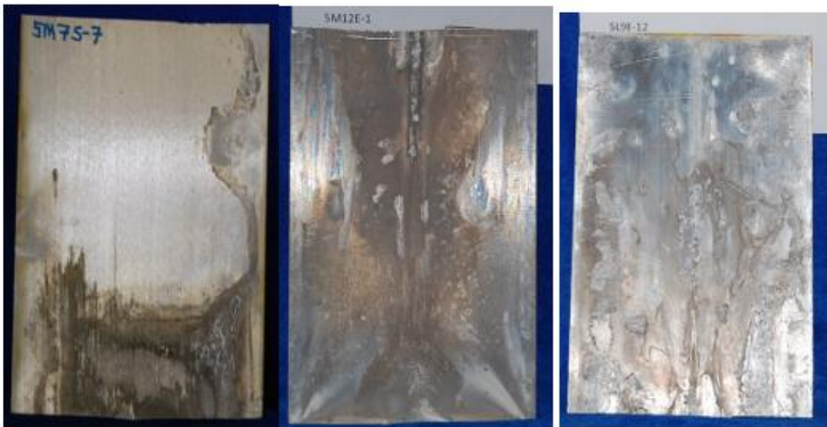
Figure 18. Back Surfaces of Region 2 Panels with Mottled and Irregular Surface Conditions
