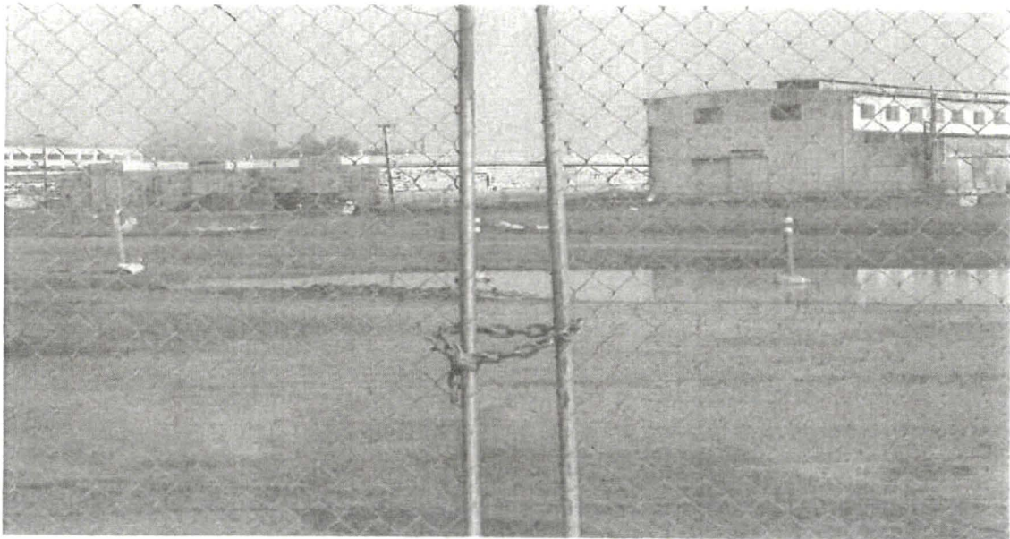
Parcel E at Radiological Screening Yard 4 (RSY4): Active RAD Waste Characterization Work Area: RAD deficiency (pad lock unsecured) as noted/corrected during end-of-day RAD integrity field check, 12.20.10
