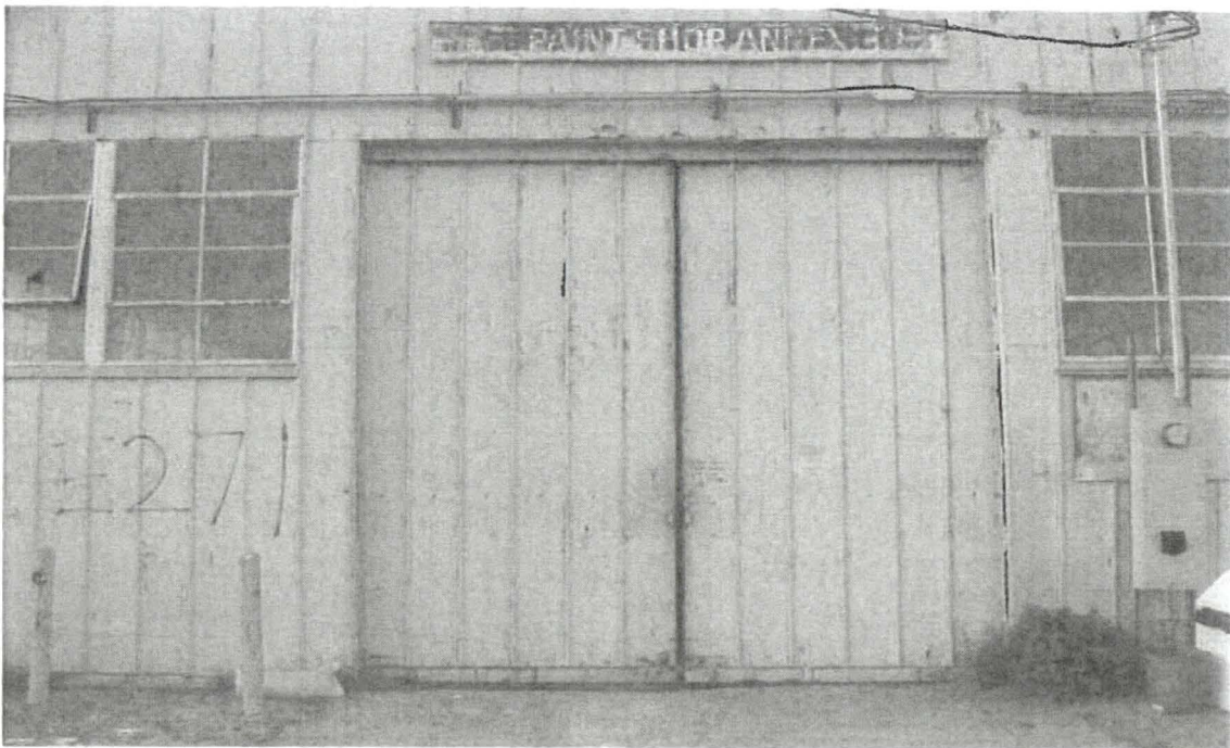
HPS Parcel B at Building 271: Active RAD Waste Characterization Work Area (View A): RAD deficiency (pad lock unsecured) as noted/corrected during end-of-day RAD integrity field check, 3.23.10
