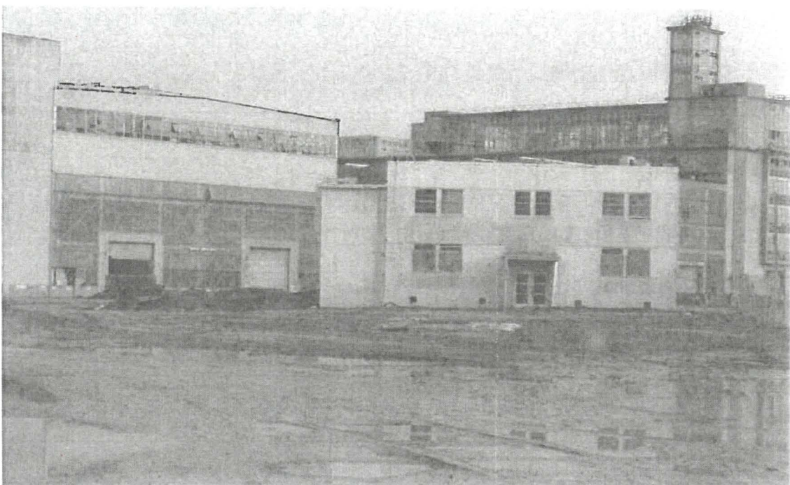
Baker Tank "Staging Area" Area as Observed: December 21, 2010
