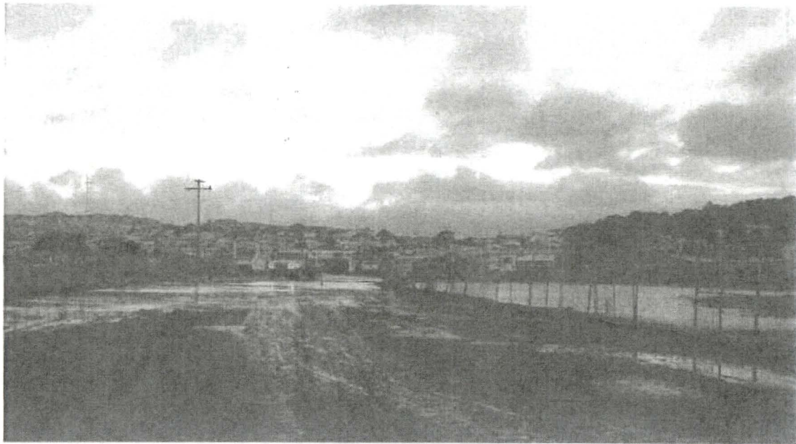
HPS Parcel E "Non-Impacted" Road: Flooded portion with Shaw vehicle stirring wake between Shaw's RCA (on left as a Radiologically Controlled Area & Contaminated Area) and Tetra Tech's RCA (on right as a Radiologically Controlled Area and Radioactive Materials Area) 12.20.10
