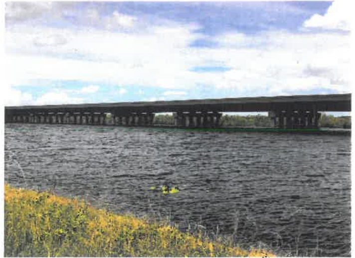
Water flowing under Tamiami Trail bridge. Photo by Susan Bennett.
