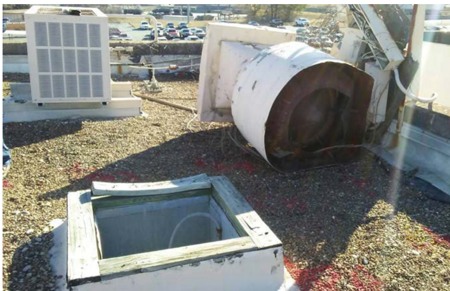
Photograph 19: Powered ventilation stack lying on roof of Cell 6.
