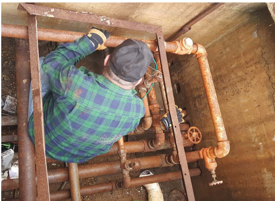
Photograph 24: Surveying the pipe chase at the east end of Cell 6.
