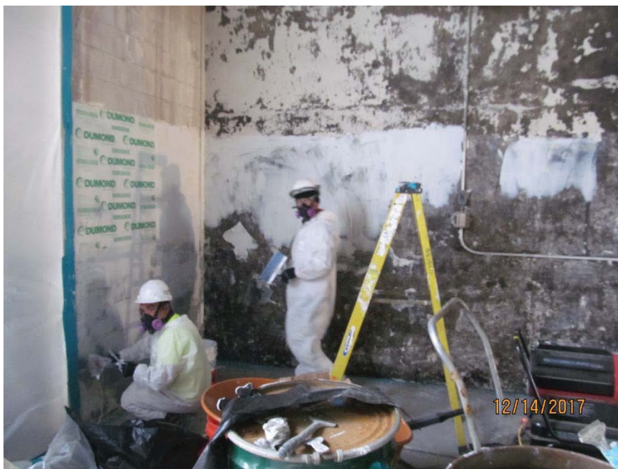
Photograph 6: Application of paint stripper in Cell 5.
