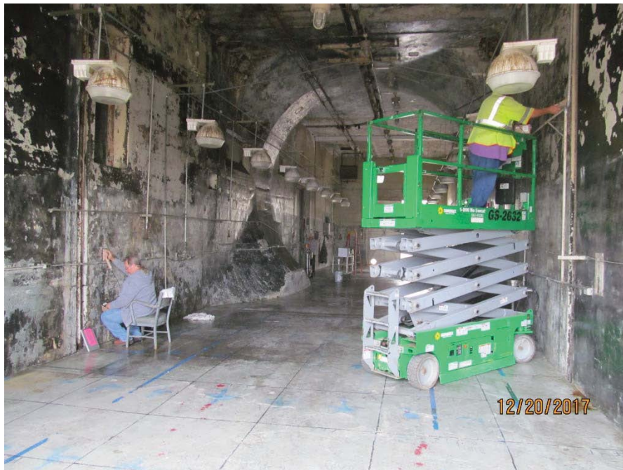
Photograph 13: Static measurements in Cell 5.
