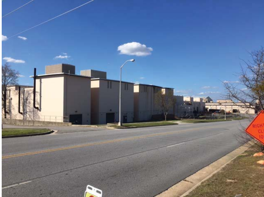
Photograph 1: View of Building 181 looking north/northwest.
