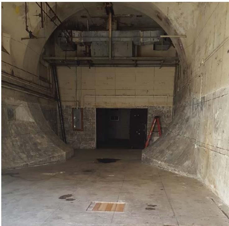
Photograph 4: Room 6A1 following removal of lead-based paint.
