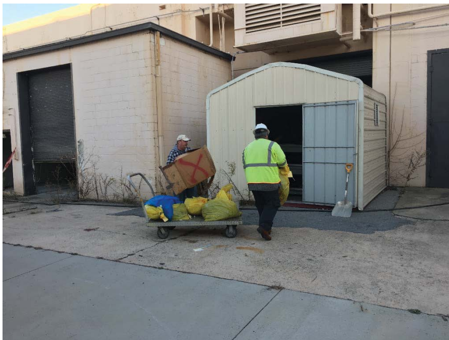
Photograph 5; Low-level radioactive waste (LLRW) storage shed outside Cell 5.
