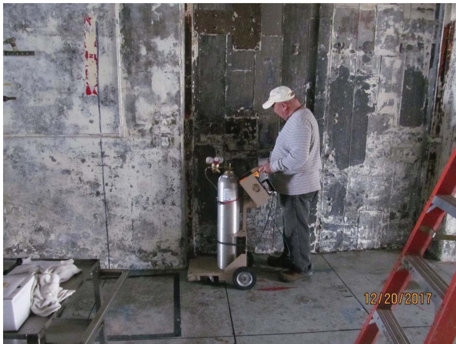
Photograph 14: Floor scanning in Cell 5.
