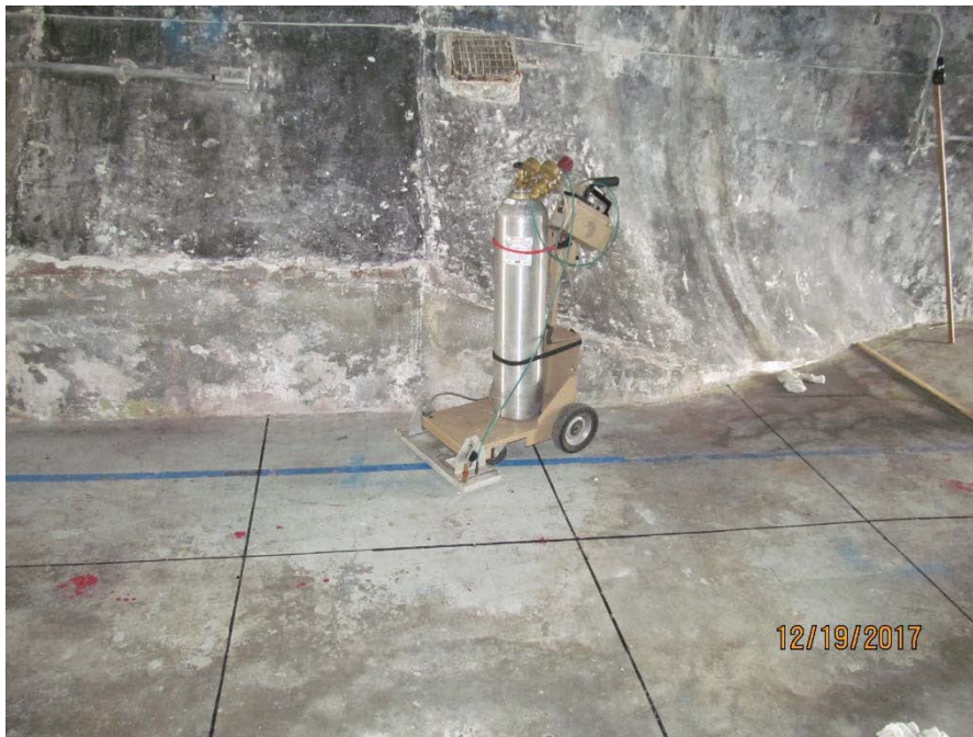
Photograph 9: Floor scanner in Room 6A1.
