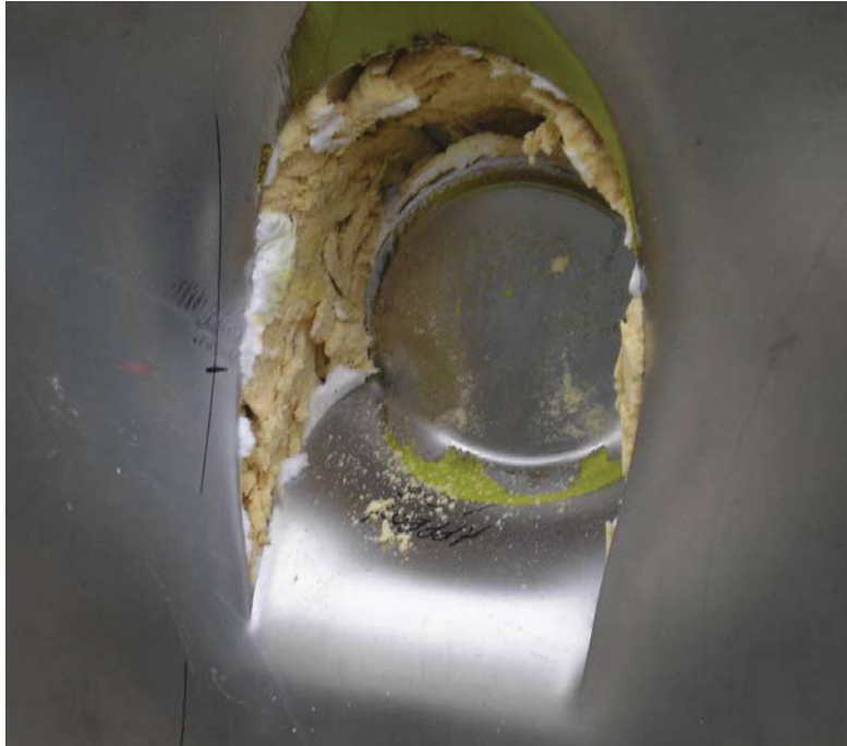
Figure 2-15 – Close-up of Puncture Damage for Test CP1
