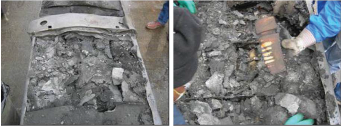
Foam Under Ceramic Fiber Paper Intumesced Filling Voids
