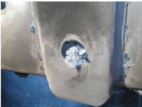
Figure 2-85 - Vent at stiffener
