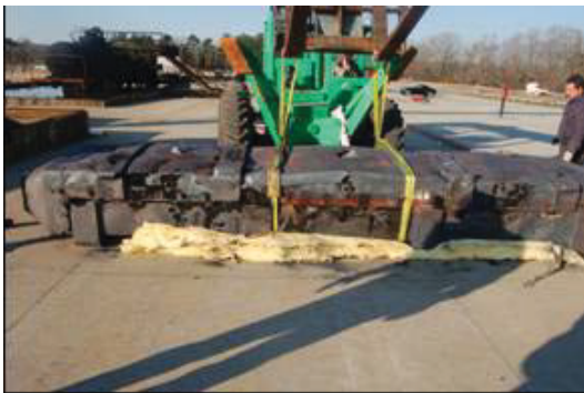
Figure 2-84 - Side view after removal from pad
