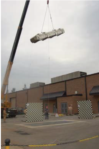
Figure 2-44 - CTU1 prior to impact
