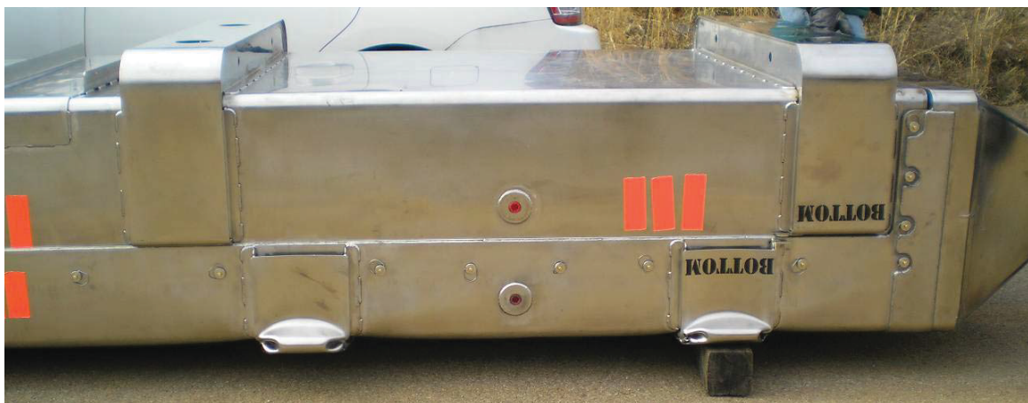
Figure 2-11 – Top End Stiffener Damage
