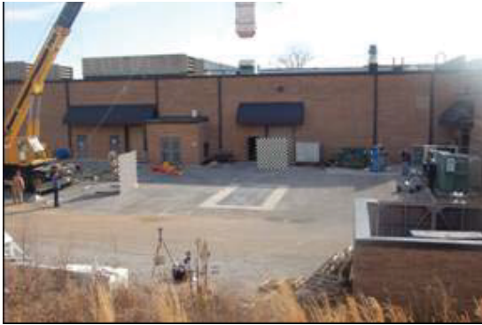
Figure 2-34 - CTU2 prior to drop
