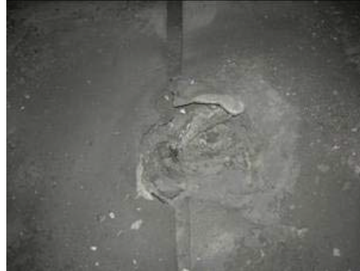
Close-up View of Puncture Bar Damage Area
