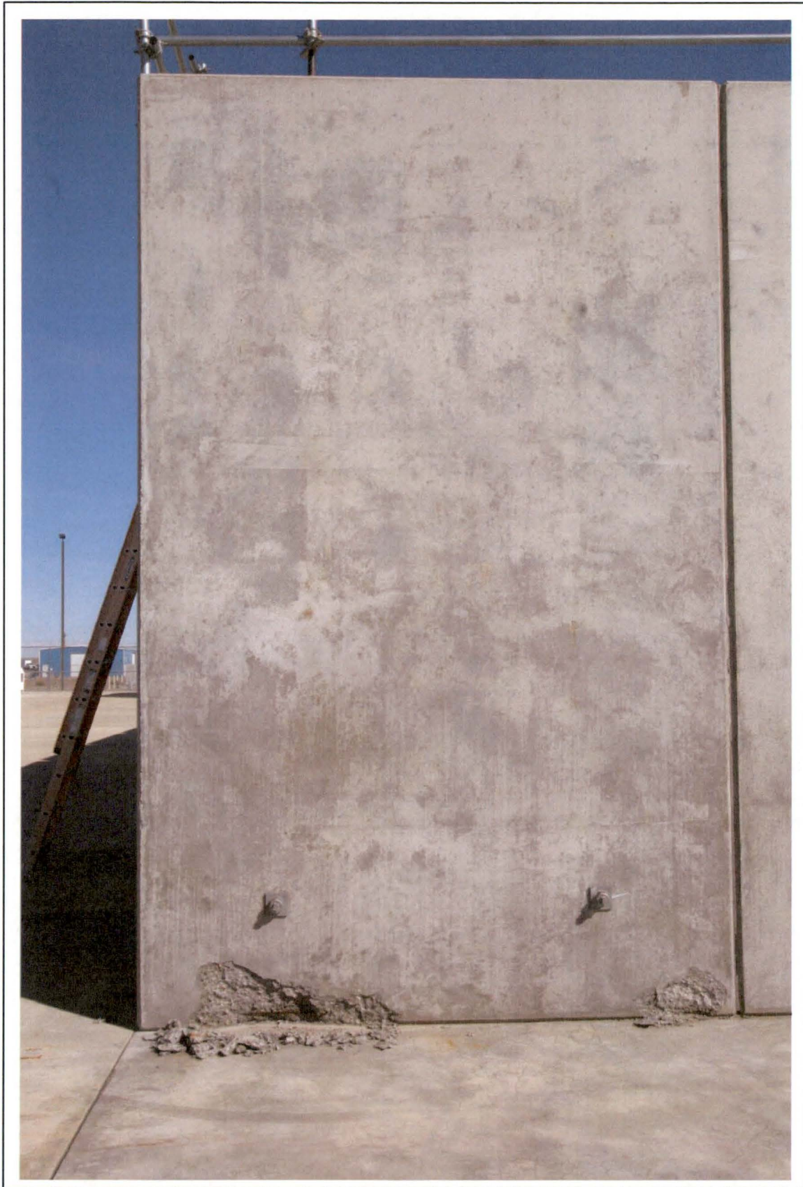
Figure 3-9: Southwest Shield Wall – Left Panel (September, 2015)
