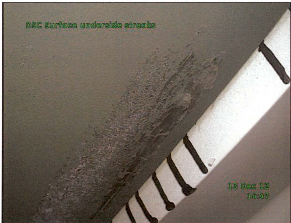
Figure 3-4: Scrape Shown on Underside of DSC S/N DOE12T-002 Inside of HSM-16 [3.11.83]
