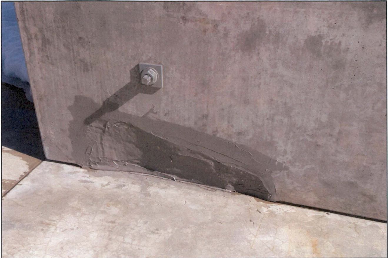
Figure 3-10: Southwest Shield Wall – Left Panel (March, 2016)
