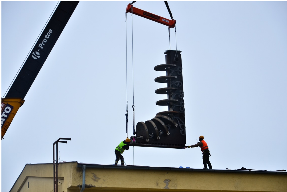
Installation – because of the dimension through the roof
