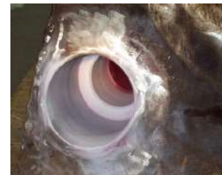
Step 3 Adapter boring, weld Prep Machining and manual PT
