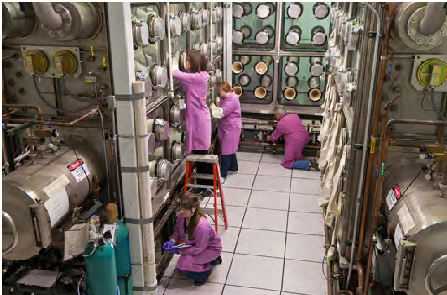
Series of interconnected inert atmosphere gloveboxes for electrochemical process development
