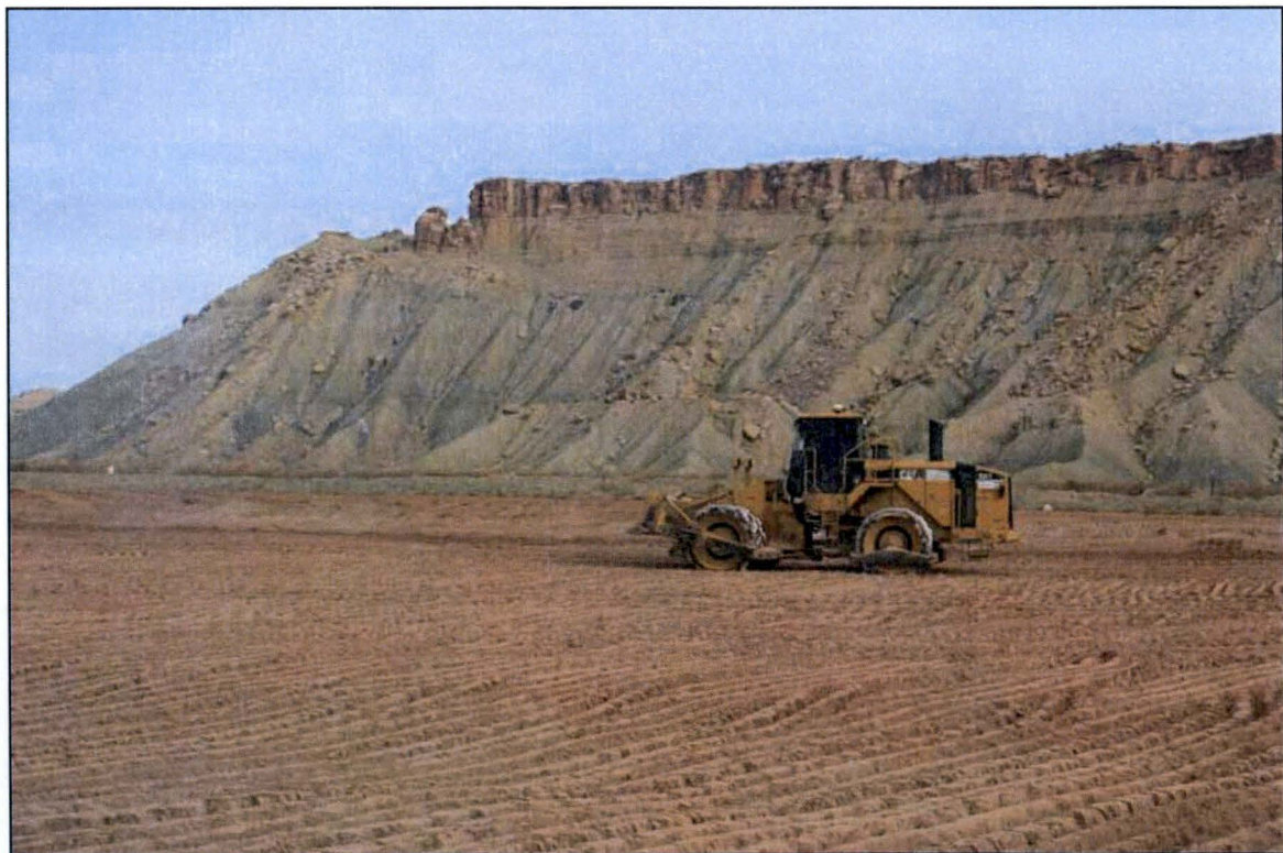
Photo 24. Sheepsfoot Scarifying Lift Area for Placement February 2018
