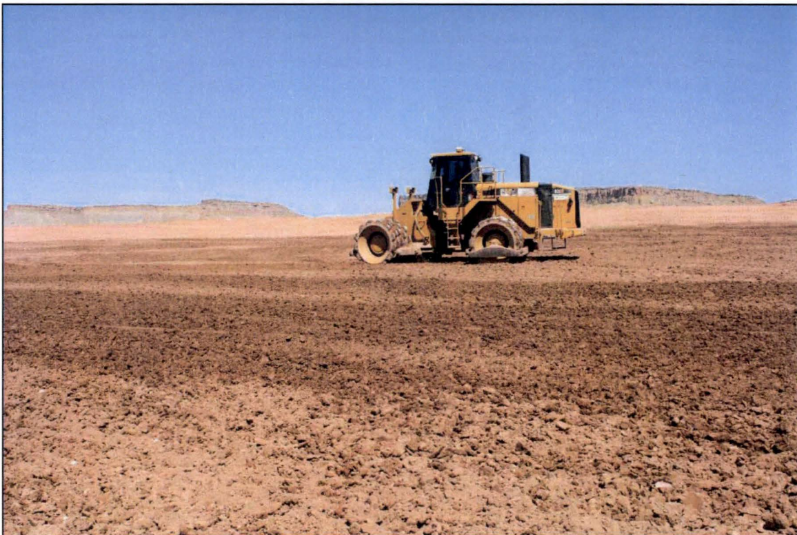
Photo 46. Compaction of Lift Area by Compactor June 2018
