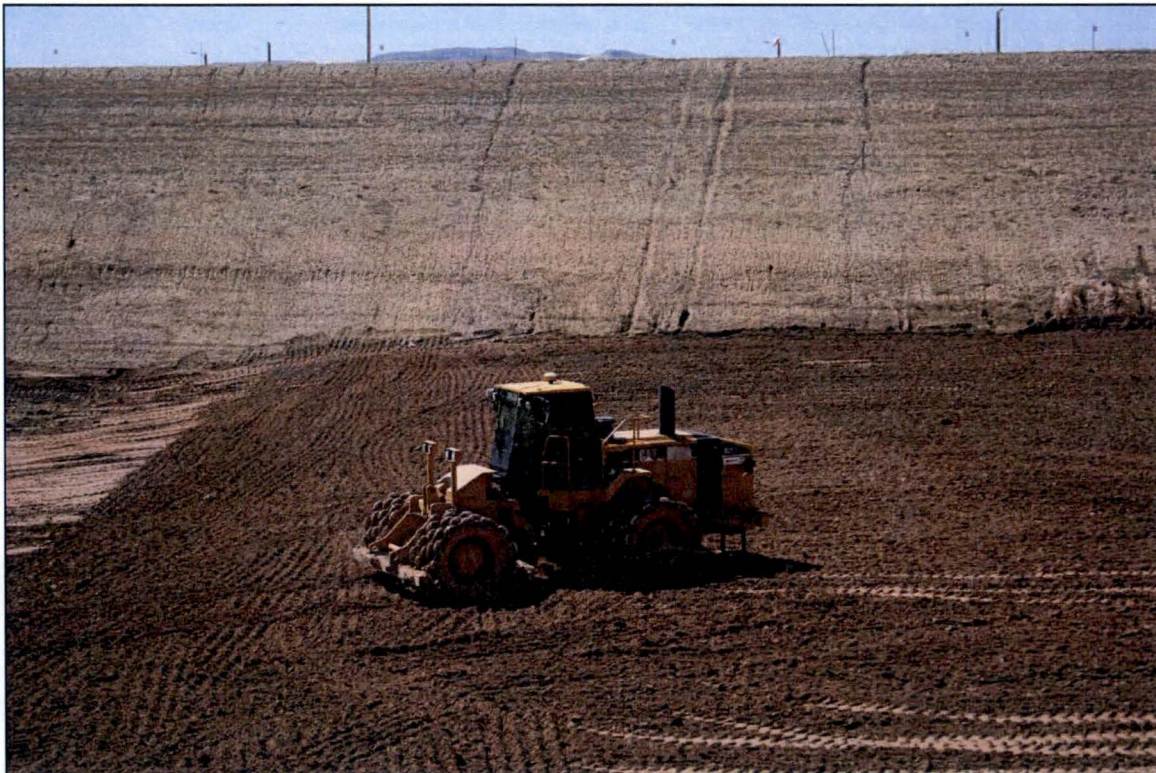
Photo 40. Compactor Compacting Lift Material May 2018
