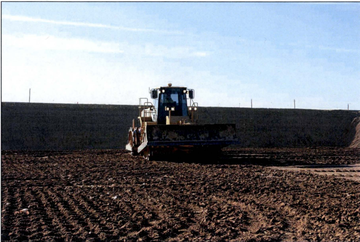
Photo 13. Compaction of Lift Area December 2017
