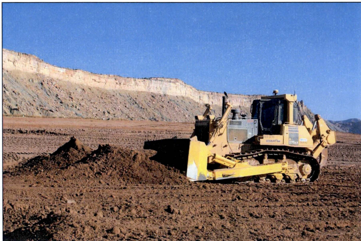
Photo 16. Dozer Placing Material December 2017
