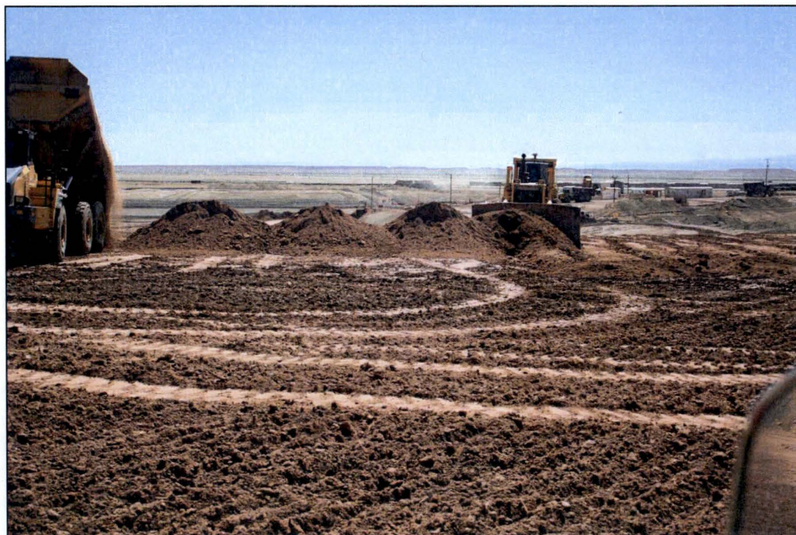
Photo 36. Dozer Placing Material on Lift April 2018
