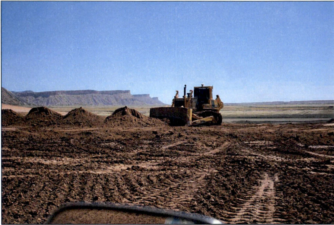
Photo 39. Dozer Placing RRM May 2018
