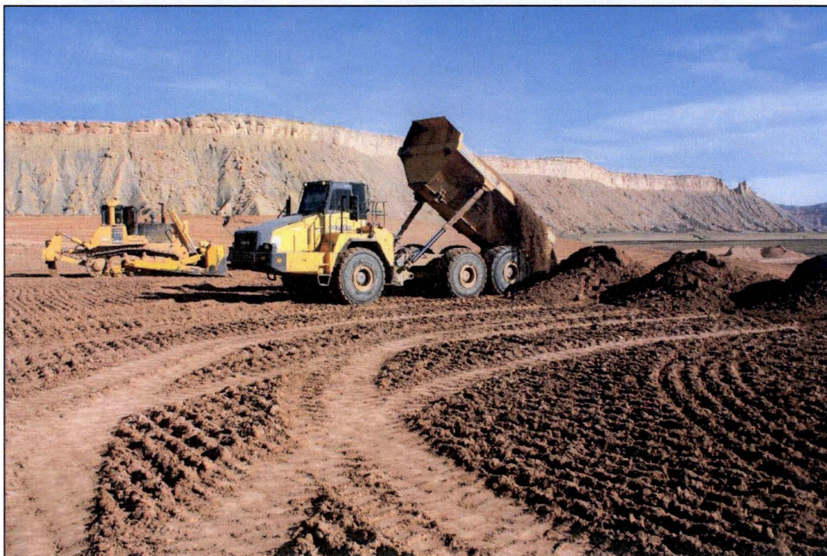
Photo 18. Truck Dumping Material on Lift Area January 2018
