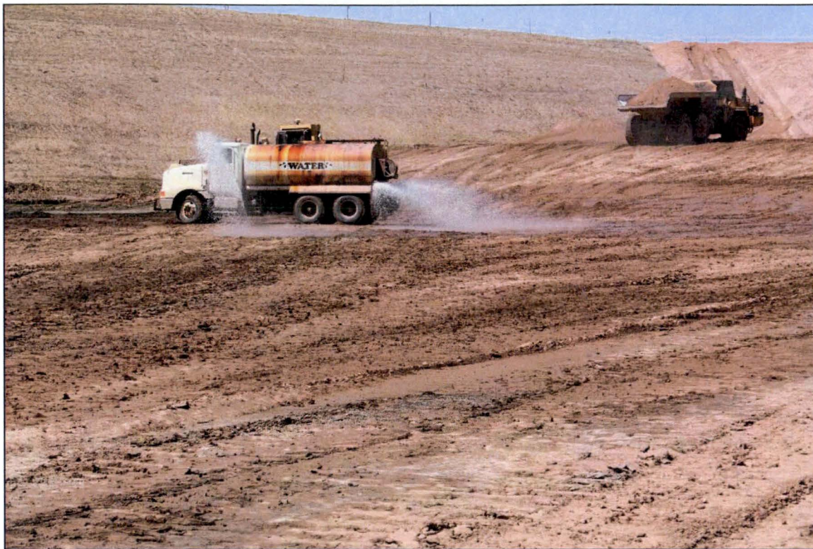
Photo 47. Watering of Cell Floor for Dust Control June 2018
