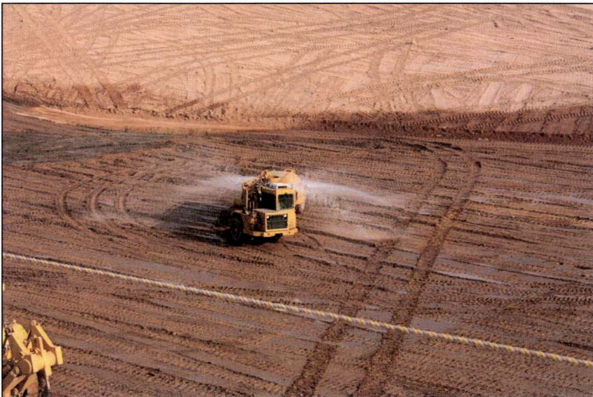
Photo 54. Watering Down of Lift Area August 2018
