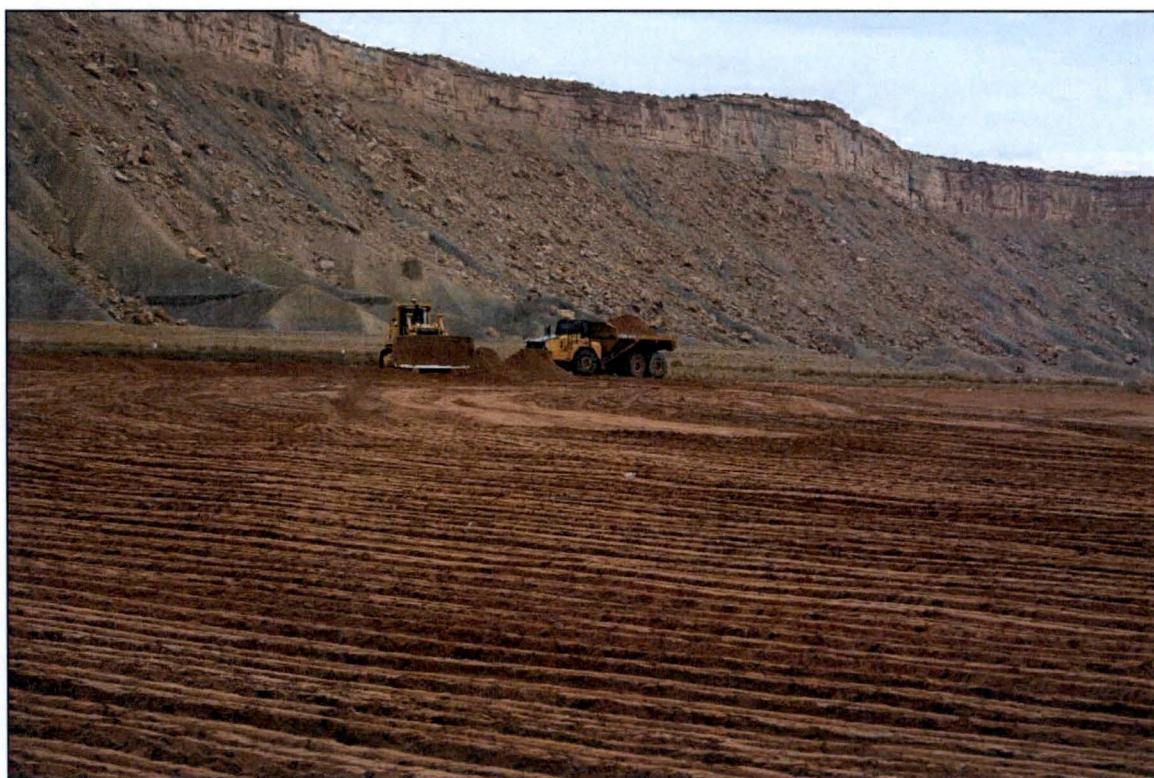
Photo 28. Dozer Placing Material on Lift Area March 2018
