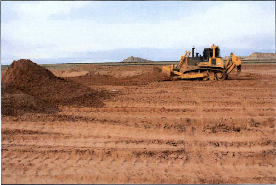
Photo 23. Bulldozer Pushing RRM for Placement February 2018
