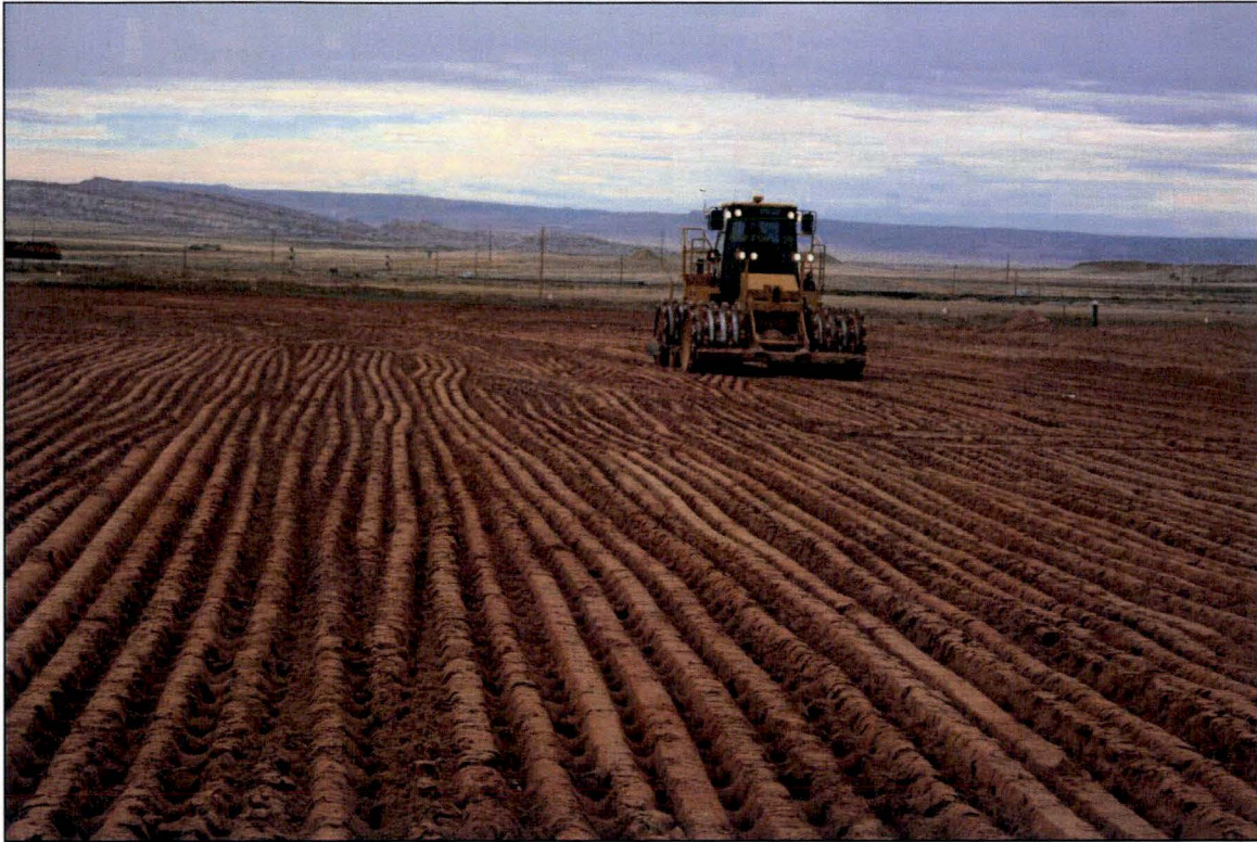
Photo 29. Compaction of Lift by Compactor March 2018
