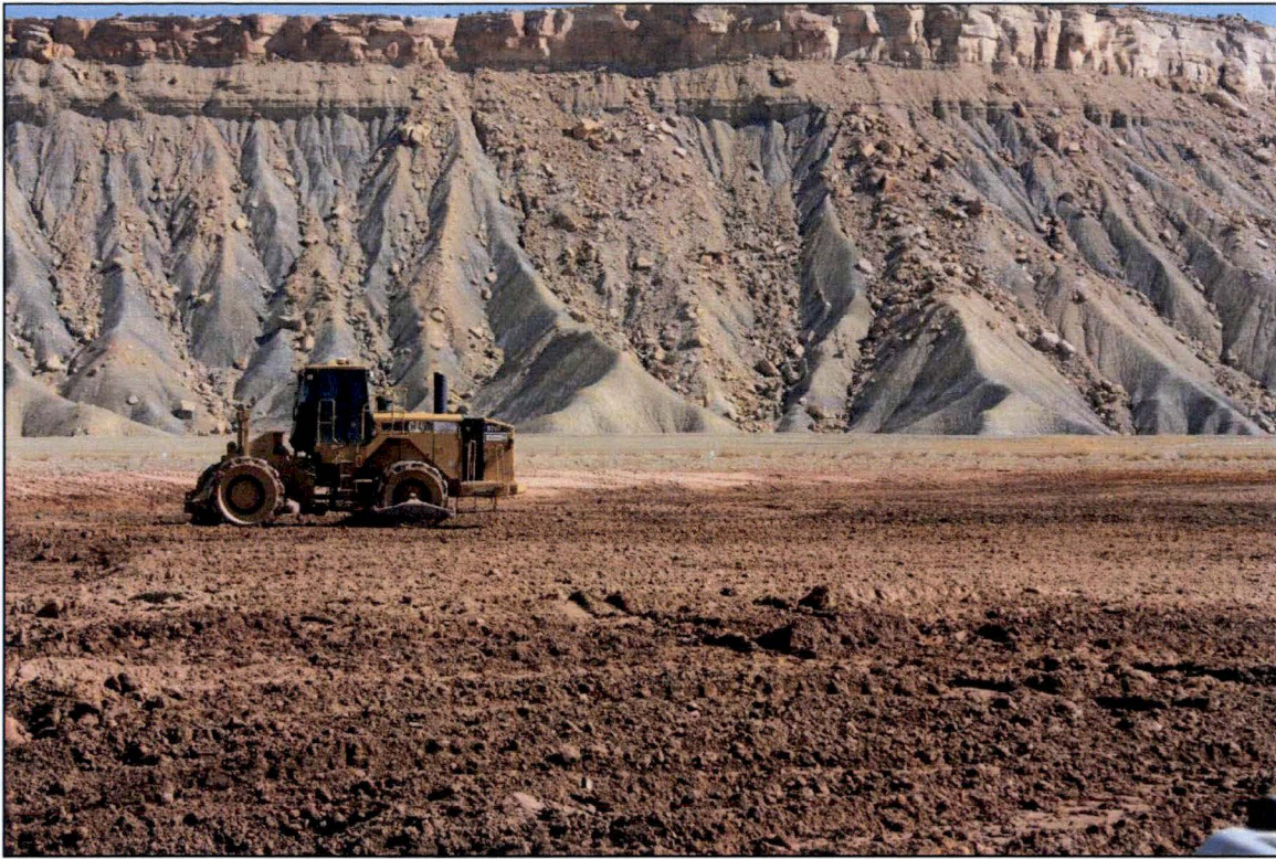
Photo 53. Compactor Compacting Material on a Lift July 2018
