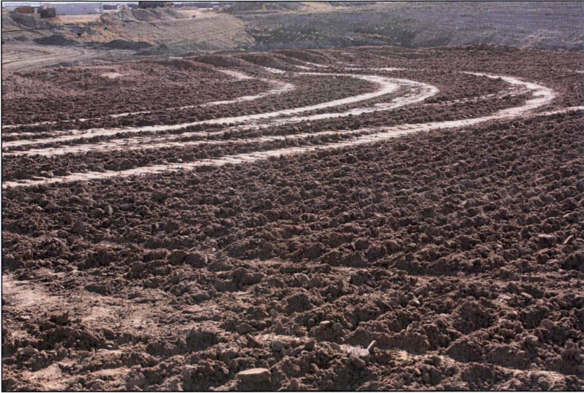
Photo 21. Compaction of Lift Area January 2018
