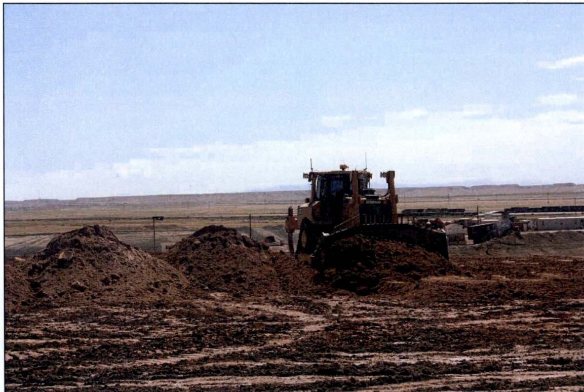
Photo 52. Placement of RRM by Dozer July 2018
