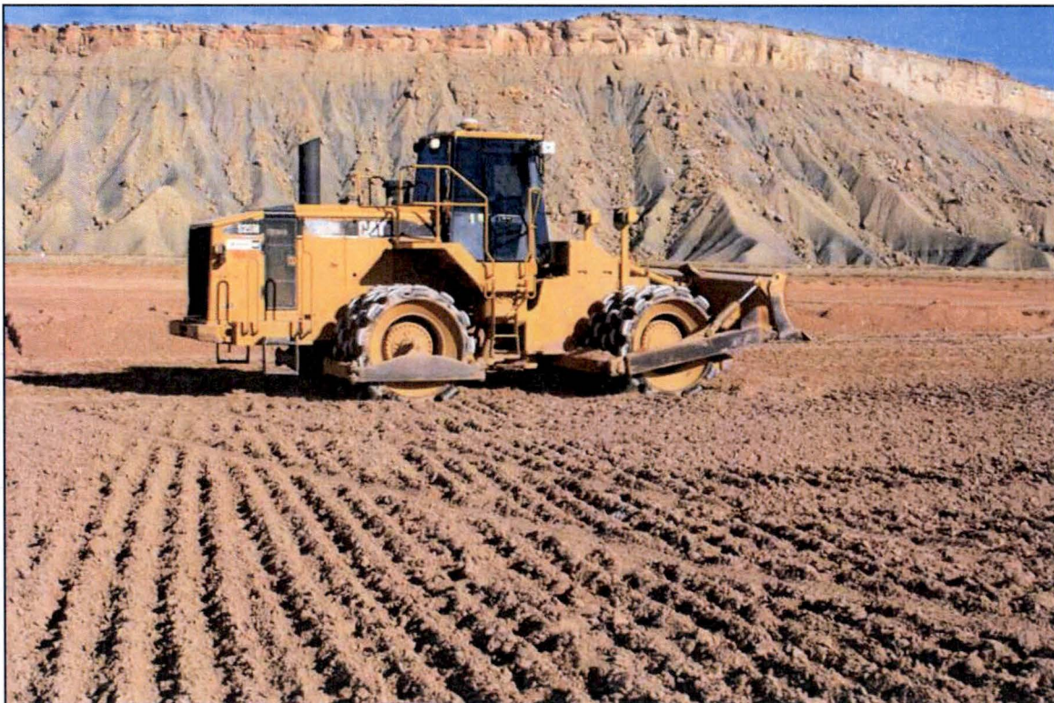
Photo 20. Scarified Lift Area January 2018
