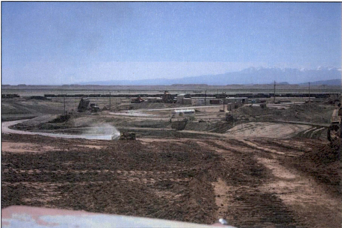
Photo 34. Water Wagon Watering Haul Routes April 2018
