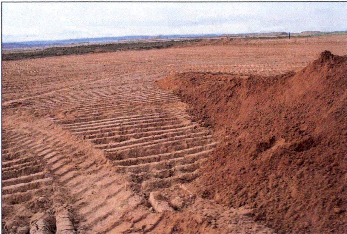
Photo 25. Underlying Lift Area Scarified for Placement February 2018
