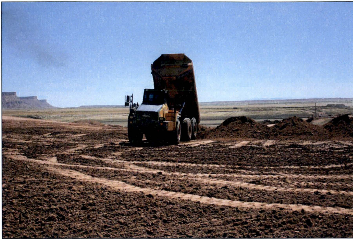
Photo 35. Haul Truck Placing Load on Lift April 2018
