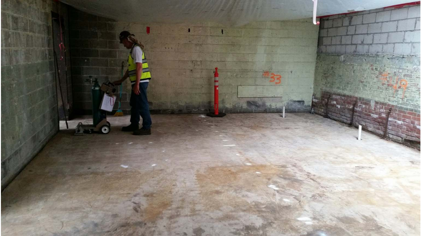
A technician performs integrated floor scans in a room on the south side of 6H.
