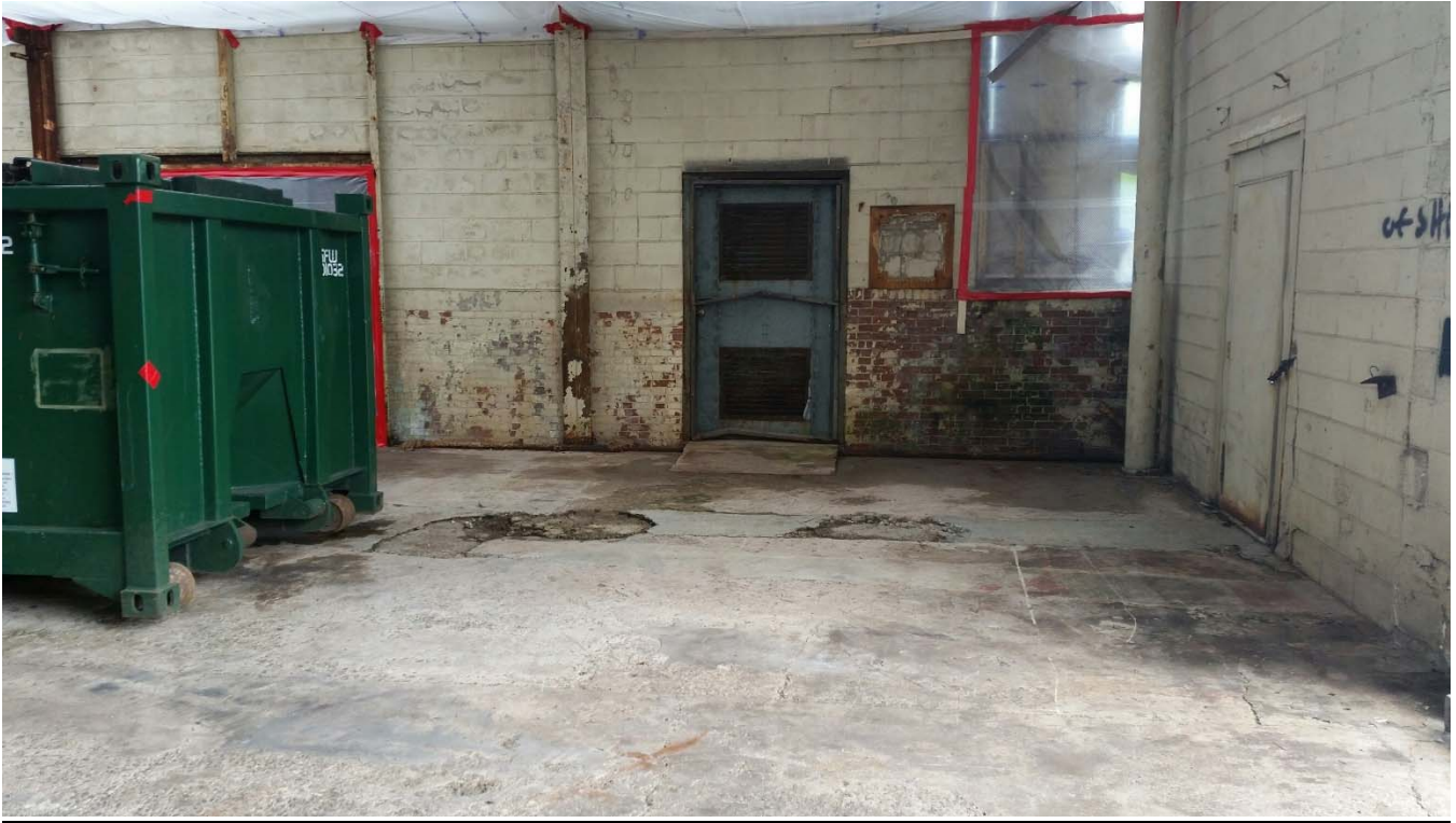
An area of 3H that was previously inaccessible to survey.
