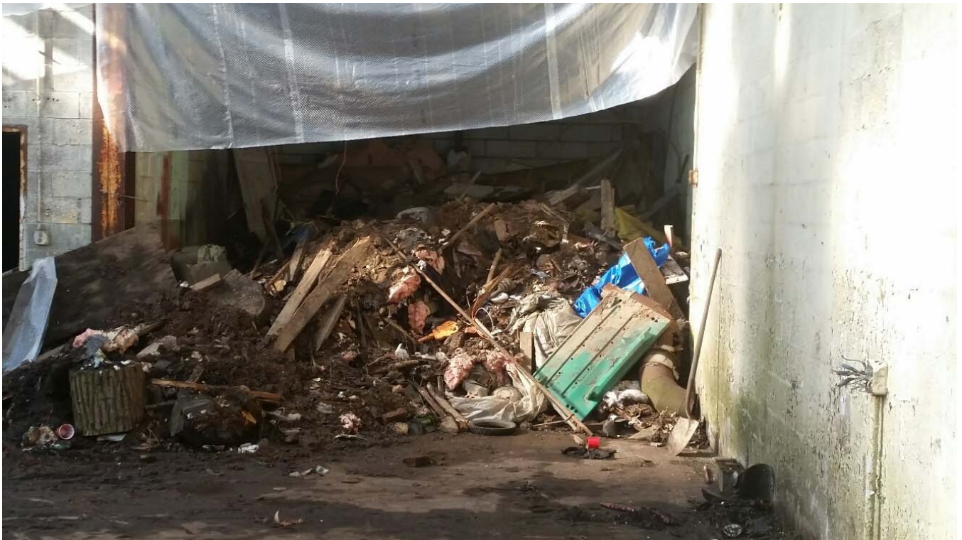
Debris piled in a side room in the east end of 3H awaiting disposal.
