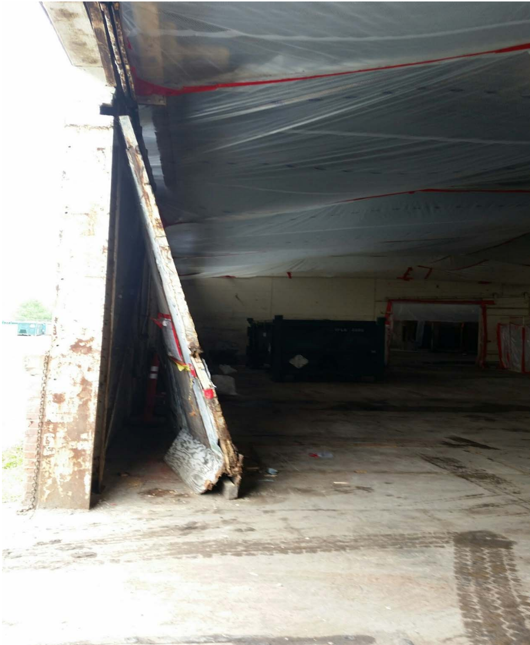
The door after contact with the truck. Bottom boards were previously broken and repaired prior to Cabrera being on-site.
