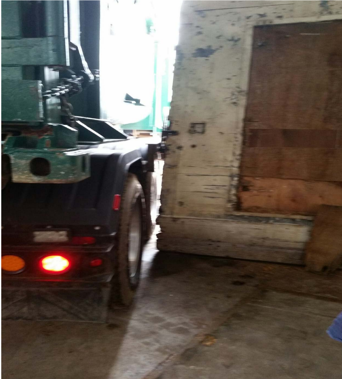
Truck after contacting the door.
