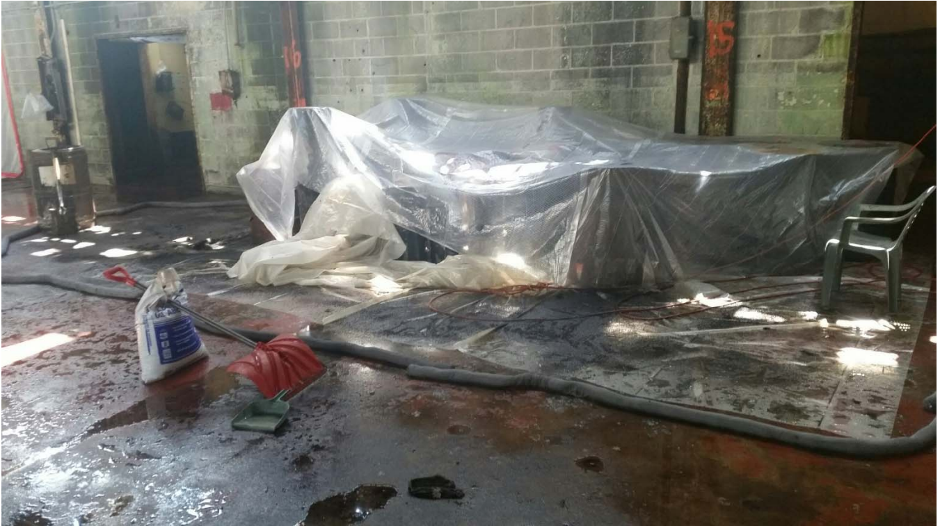
Cleanup of leaking drum in bldg. 6H. The area was surrounded with absorbent booms and dried.
