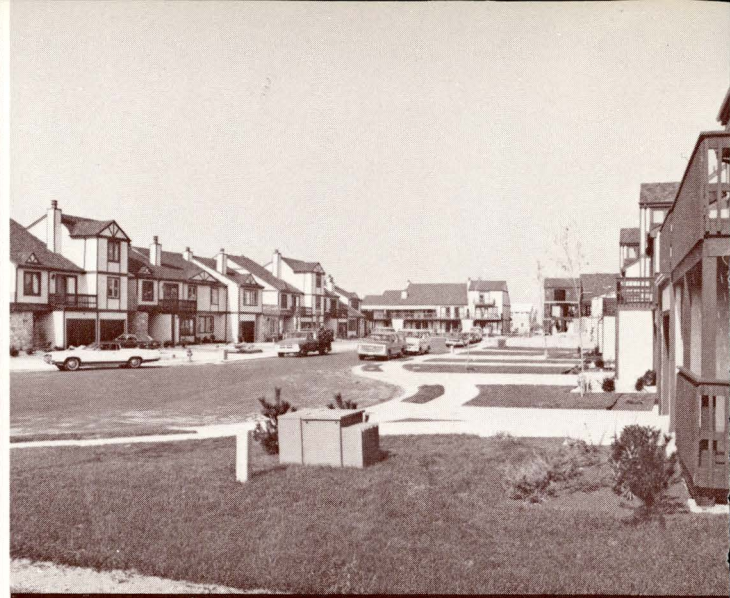
The Company is providing complete underground service to the stylish Beacon Beach condominiums in Brigantine. The condominiums are equipped with electric heat pumps.
