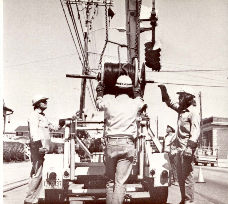
A "cable pulling" job was the order of the day for this overhead line crew in Sea Isle City.
