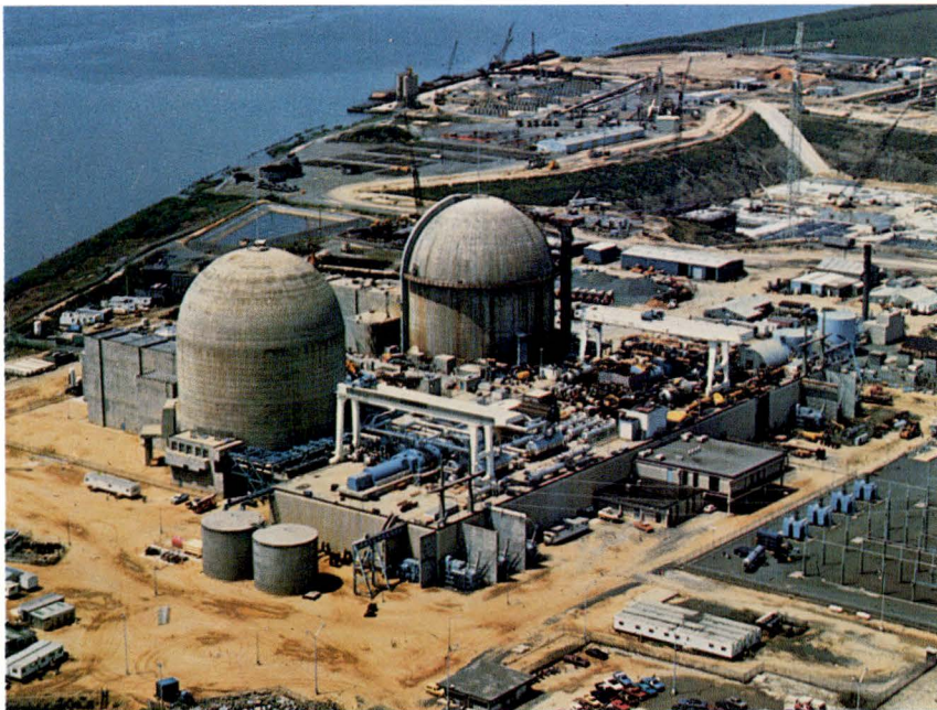
The Salem Generating Station Unit #2 was 85% complete at year end and when put into commercial operation in mid-1979, will raise the station's capacity to 2,200,000 kilowatts. The Hope Creek site can be seen at top of photo.
