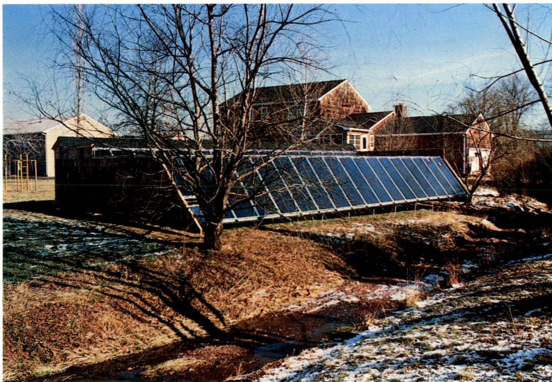
These two banks of solar panels will be used to help provide heat and hot water for the home shown in background. This is part of PSE&G's three-year program to test solar water heating, space heating and pool heating systems in customers' homes.
