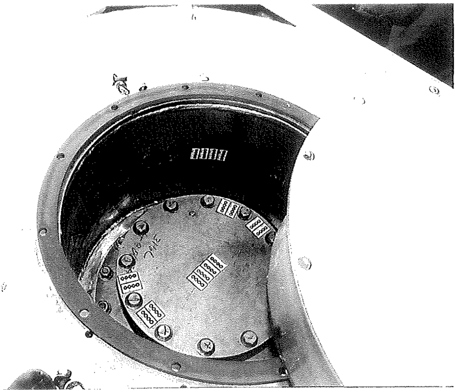
Figure A-14. Installation of Thermal Indicator Tapes Within the Lid Opening.
